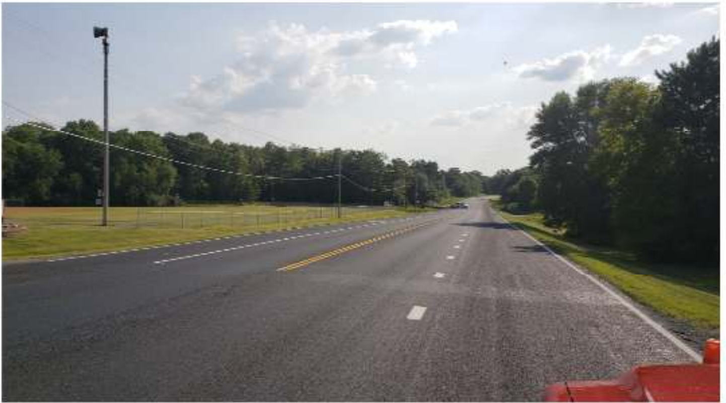
New Road Markings
