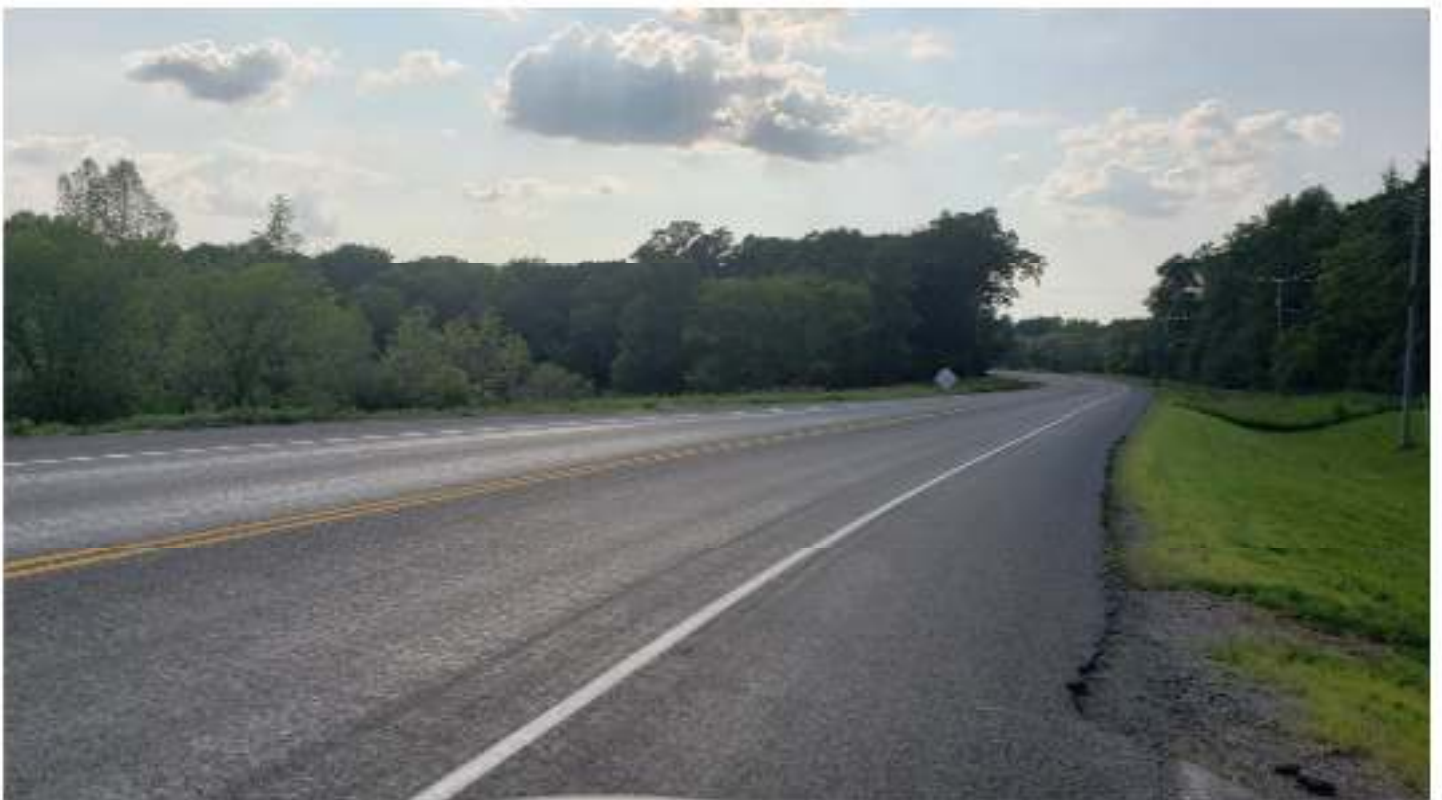
New Road Markings
