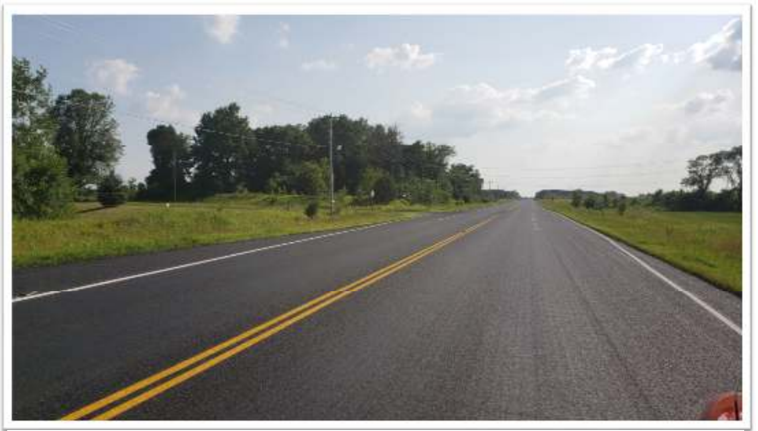
New Road Markings
