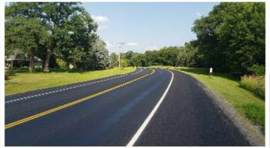
New Road Markings
