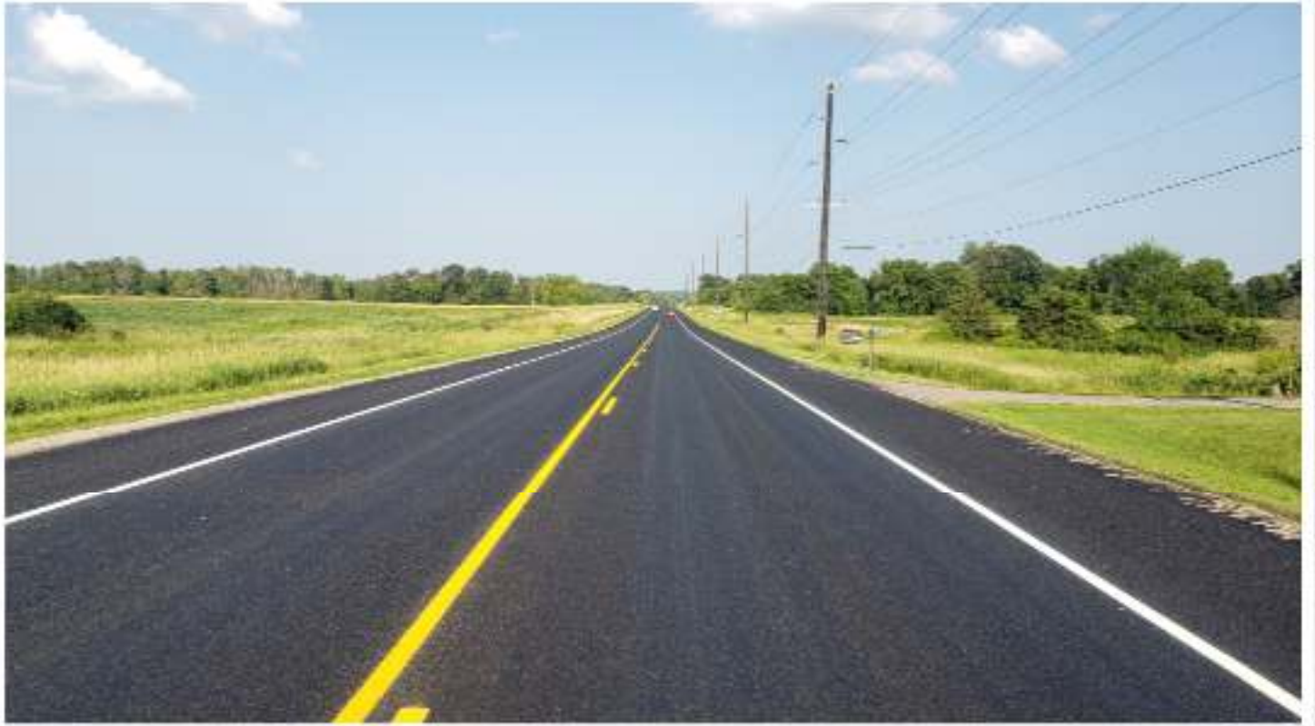
New pavement markings
