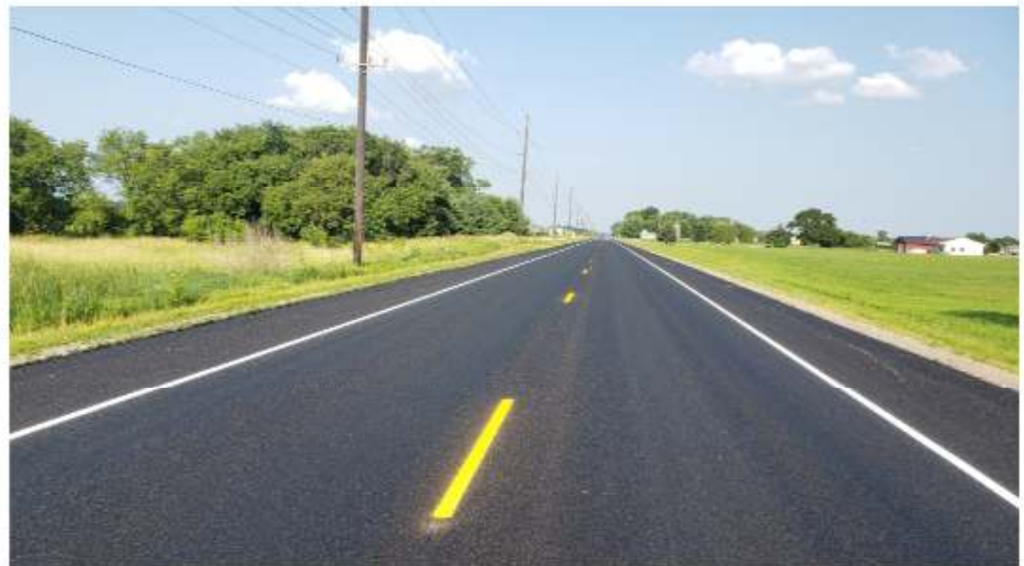
New pavement markings
