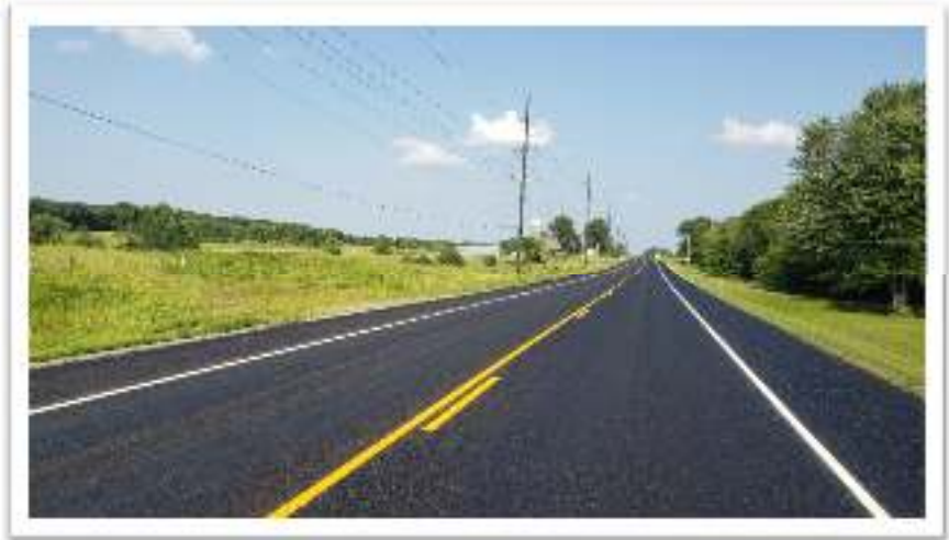
New pavement markings
