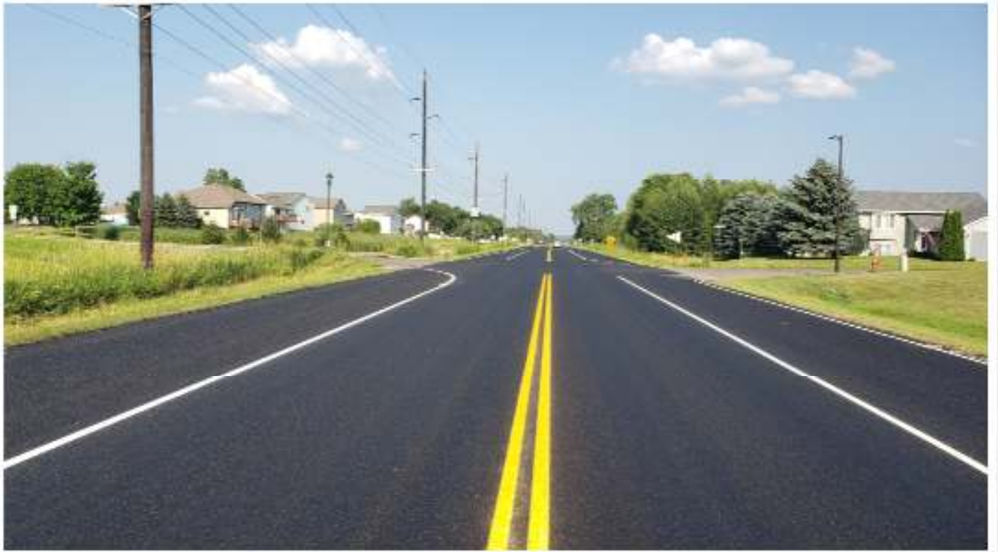
New pavement markings
