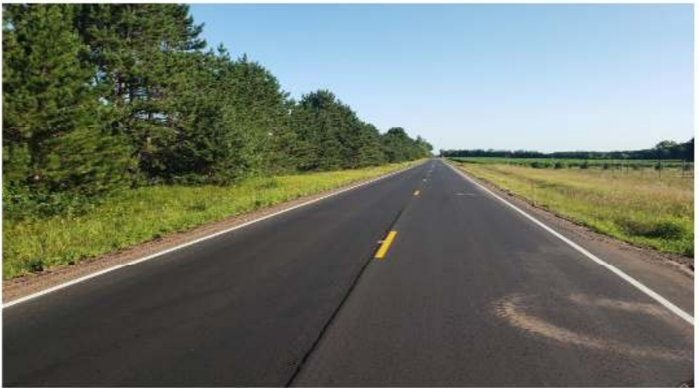
New pavement markings
