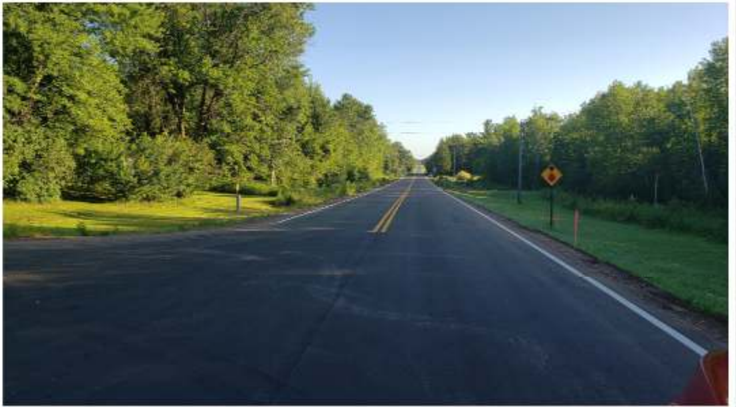
New pavement markings
