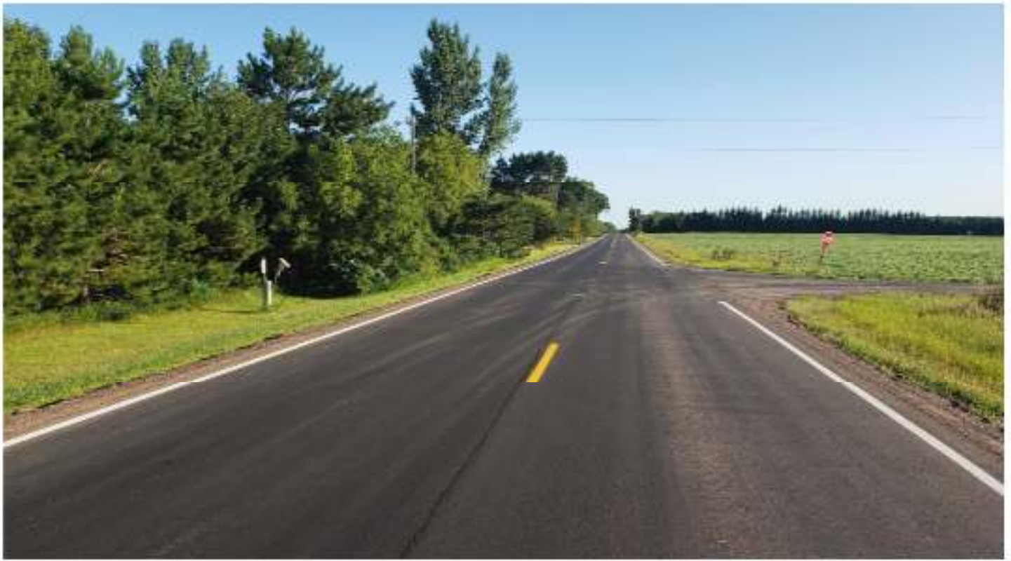
New pavement markings
