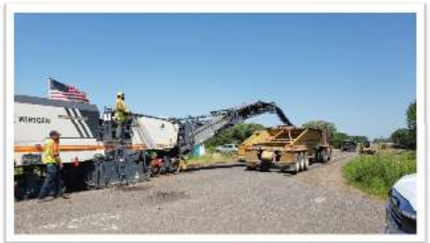
Reclaiming machine at work
