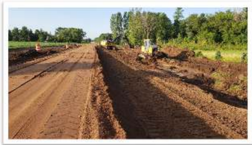
Subcutting existing road bed.
