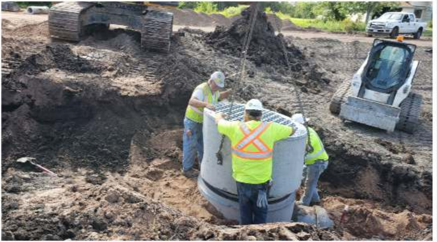
Installing new concrete culverts
