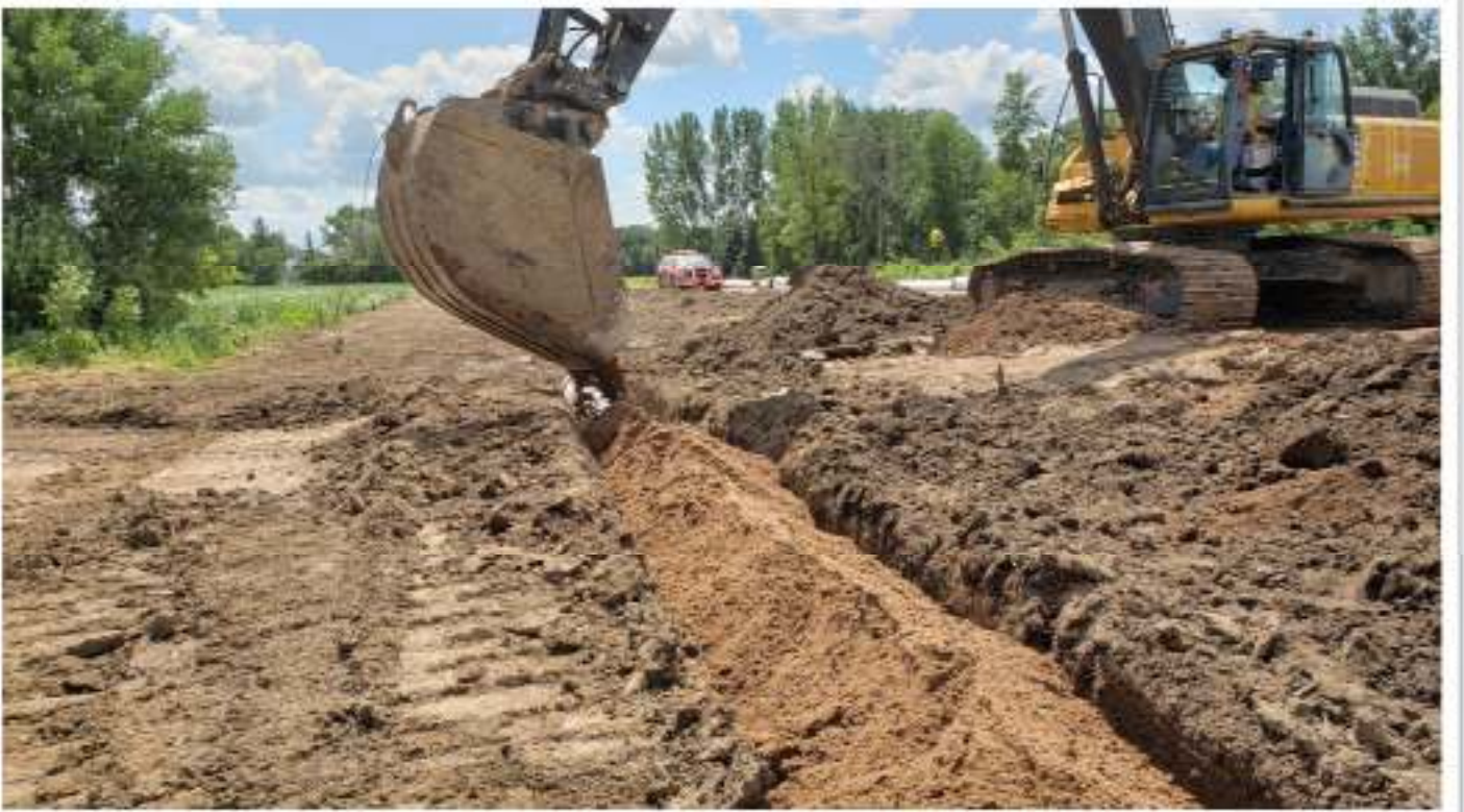
Backfilling new culvert
