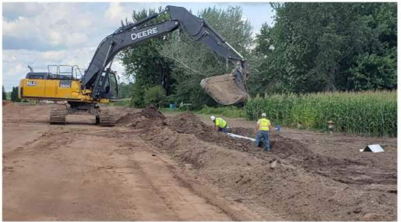
Placing new pipe culverts
