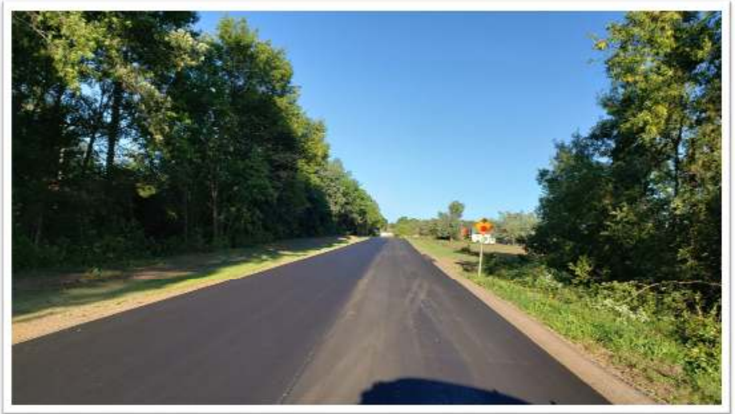
County Road 59 new pavement
