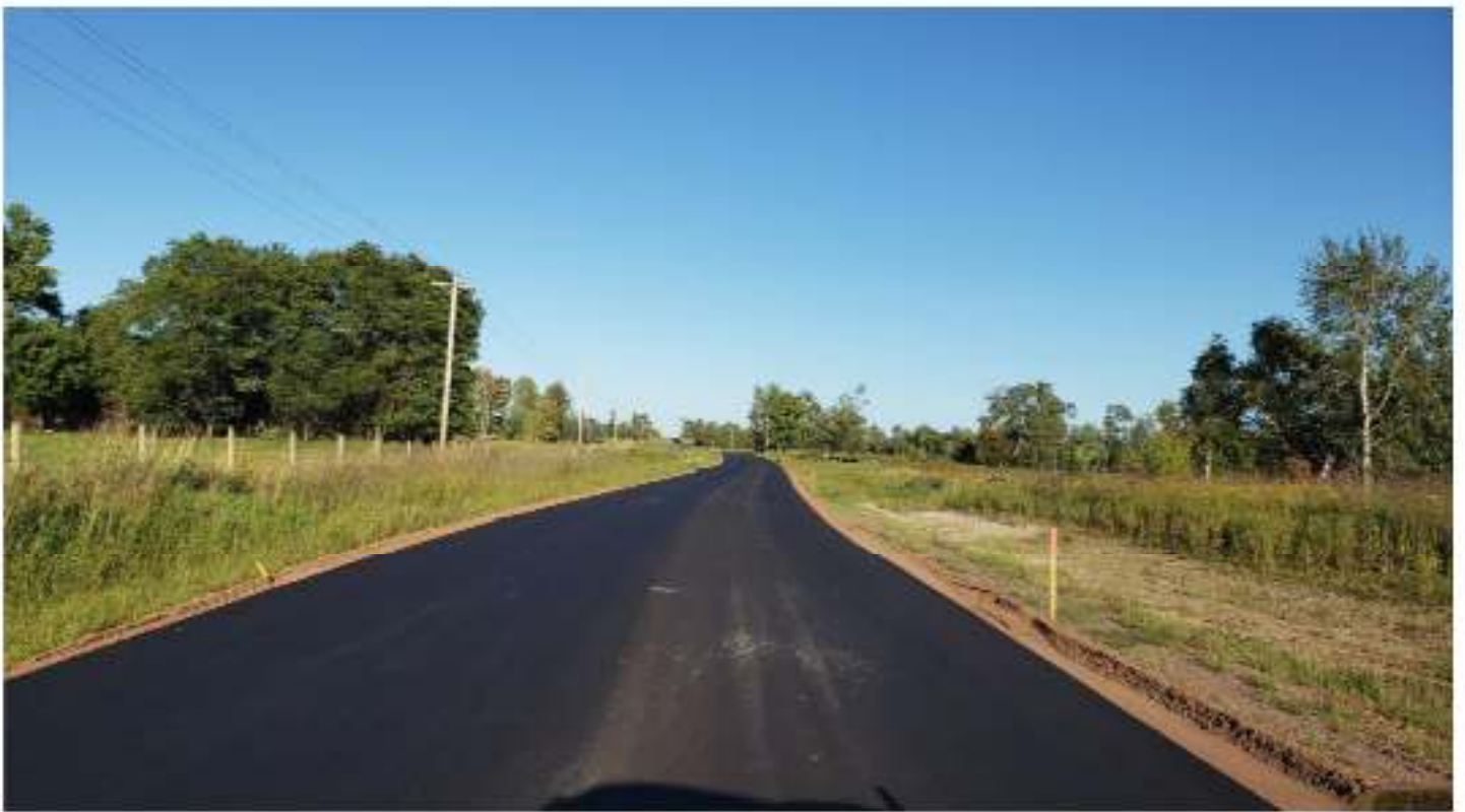
County Road 59 new pavement
