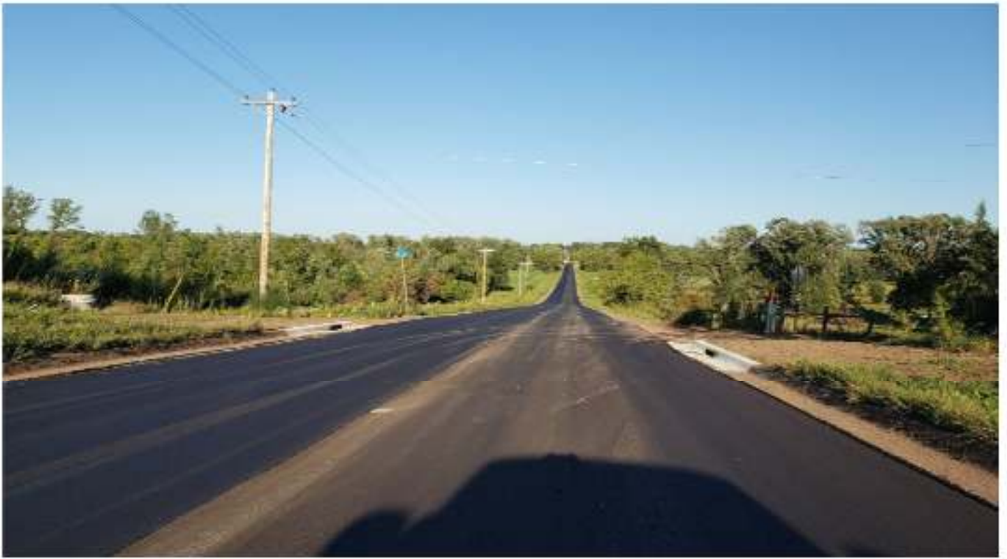
County Road 59 new pavement
