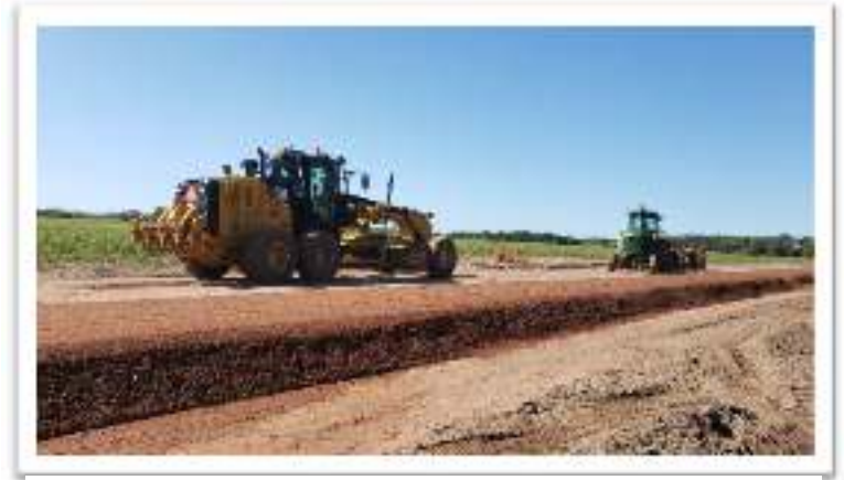
Placing new gravel
