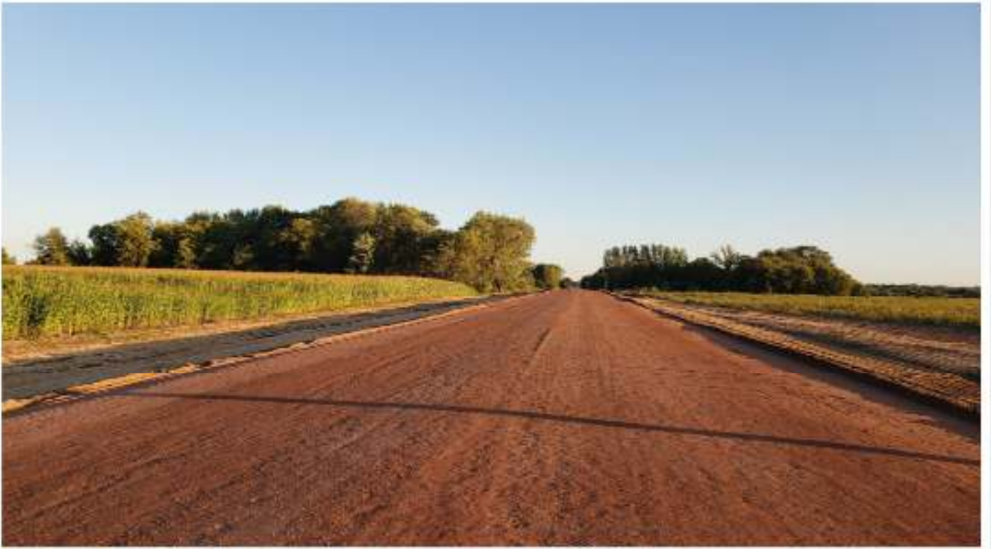
Finished gravel prior to paving
