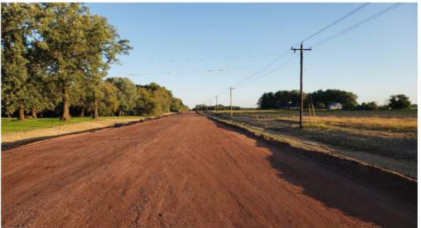
Finished gravel prior to paving
