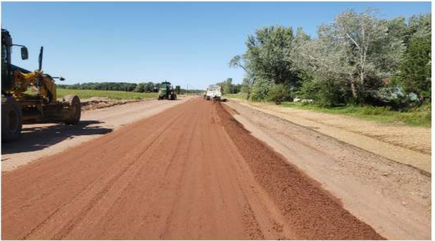
Placing new gravel
