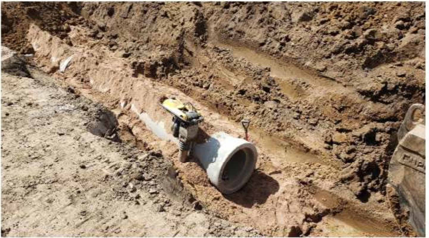
Storm sewer installation
