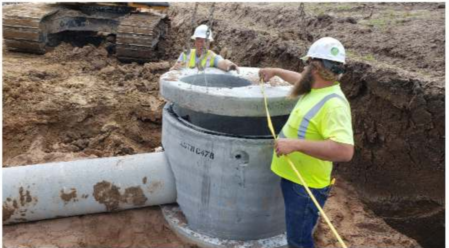
Setting a new drainage structure
