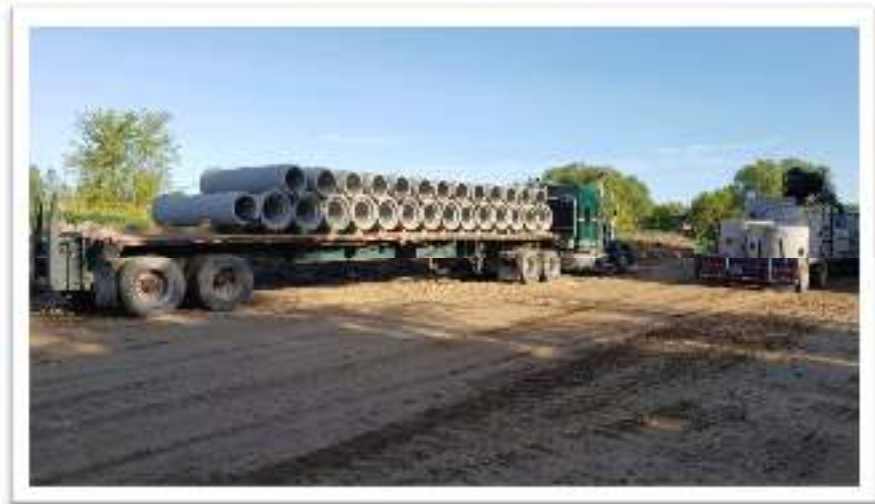
Storm sewer pipe being delivered
