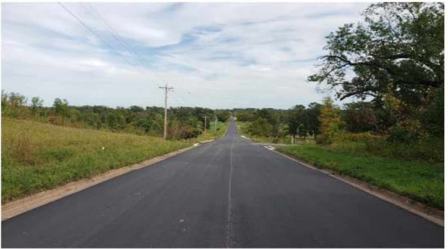
County Road 59 new pavement
