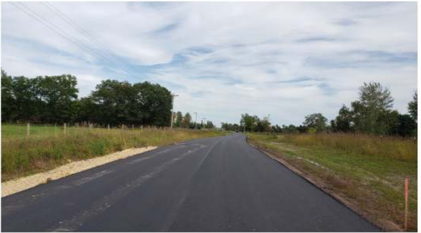
County Road 59 new pavement
