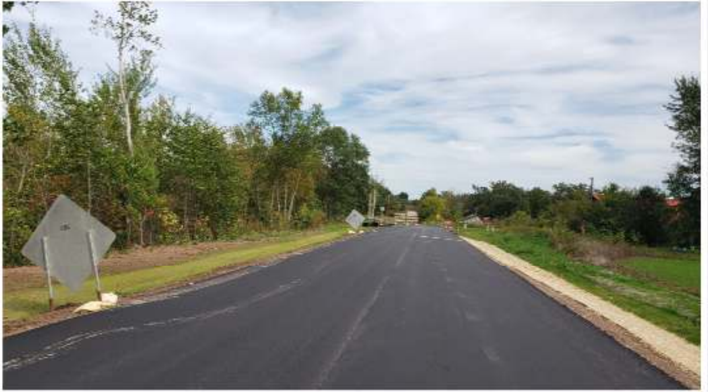
County Road 59 new pavement
