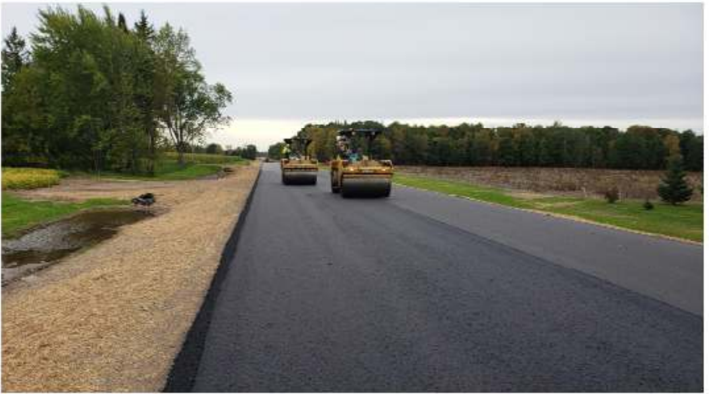
Pavement rollers at work
