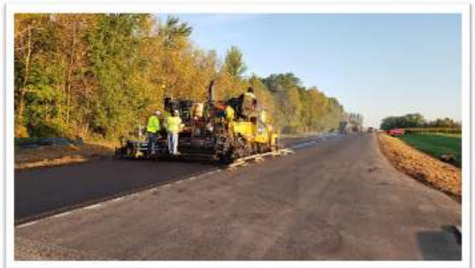
Paving final layer
