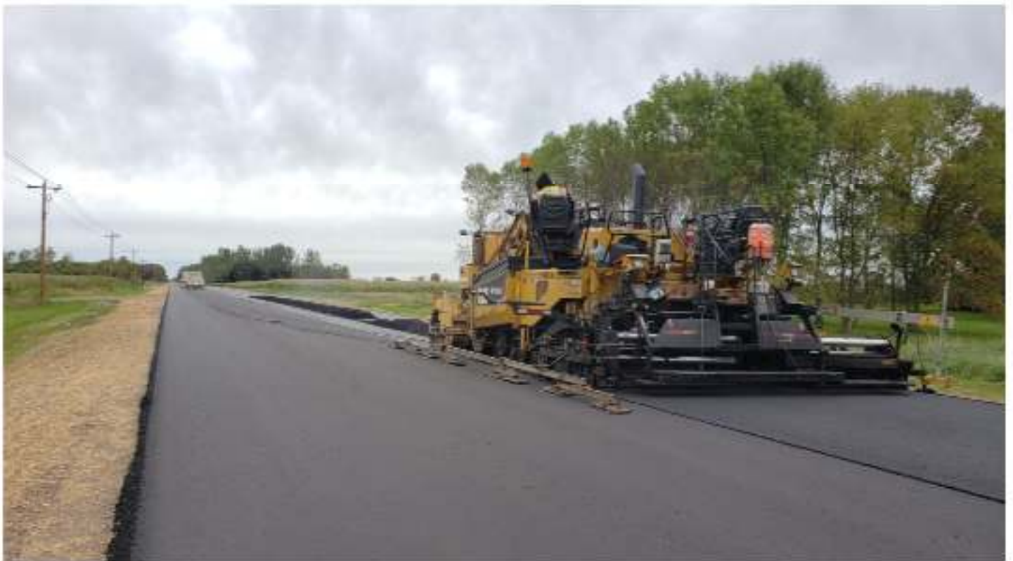
Paving final layer
