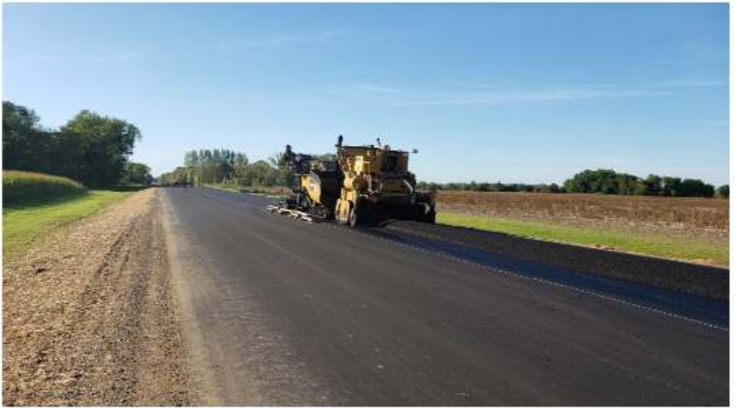
Paving final layer
