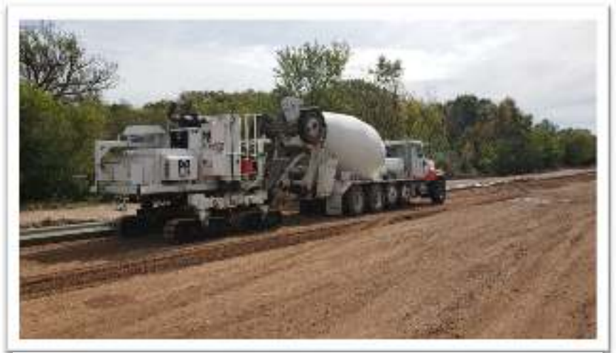
Placing Concrete Curb and Gutter
