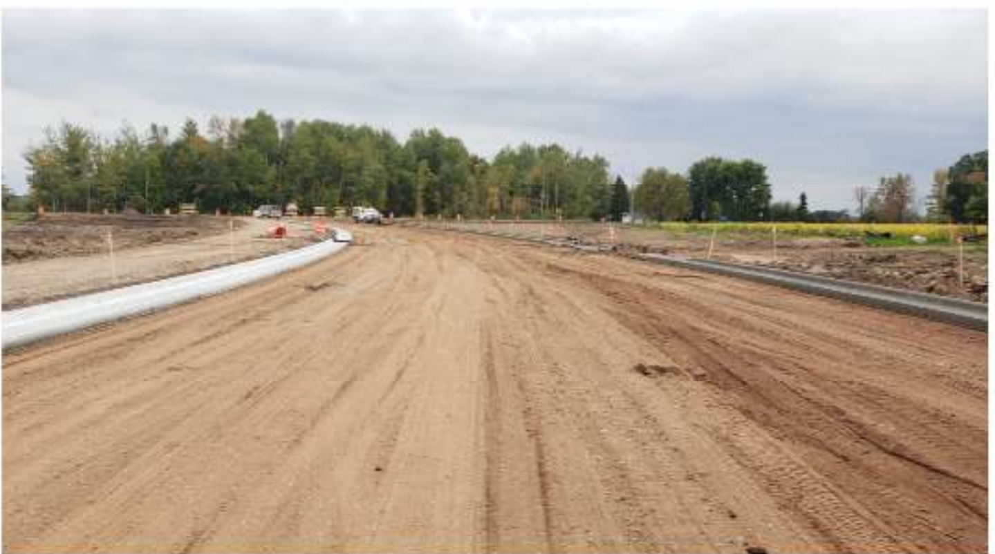
Placing Concrete Curb and Gutter
