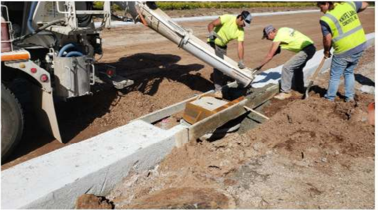
Pouring new concrete catch basins
