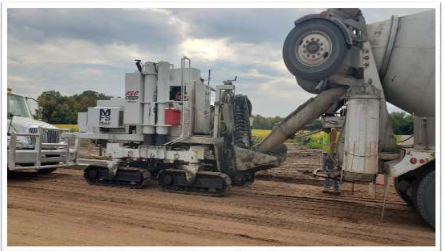
Placing Concrete Curb and Gutter
