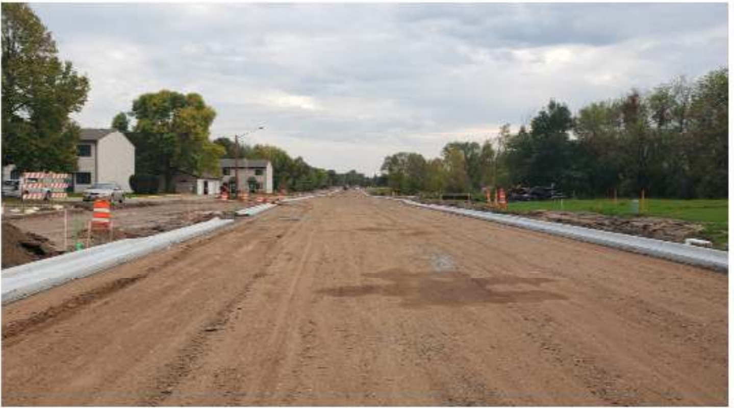
Placing Concrete Curb and Gutter
