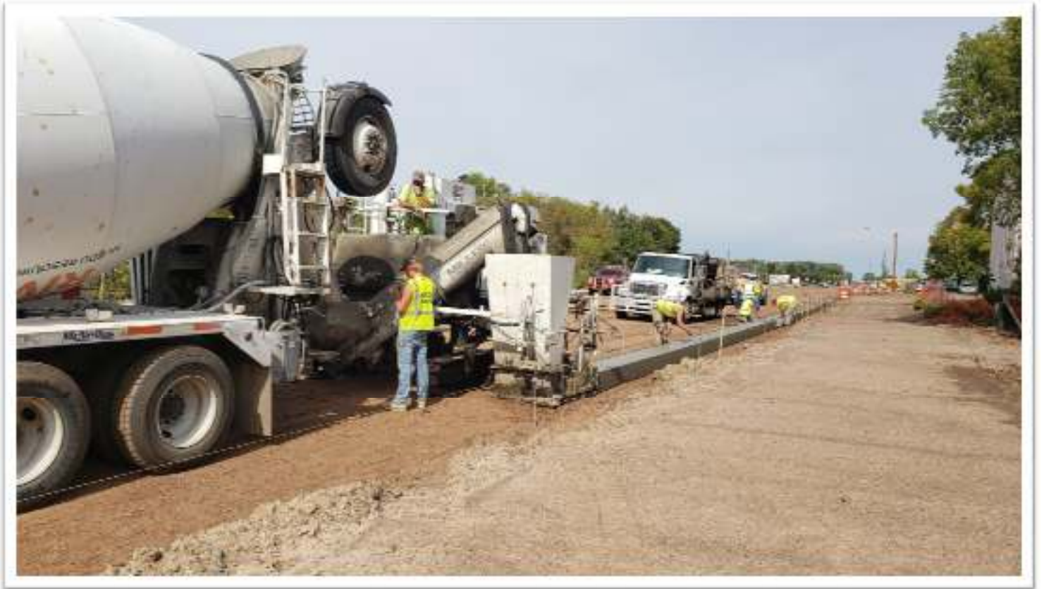
Placing Concrete Curb and Gutter
