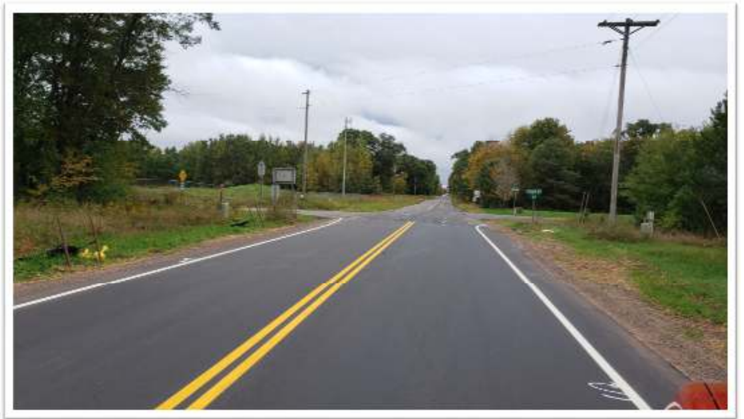
County road 78 completed
