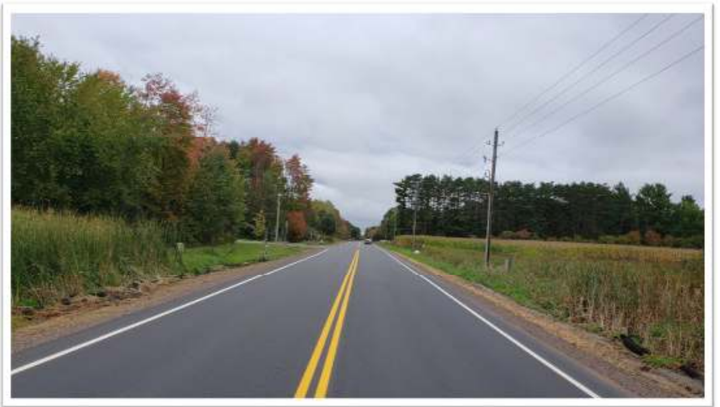
County road 78 completed
