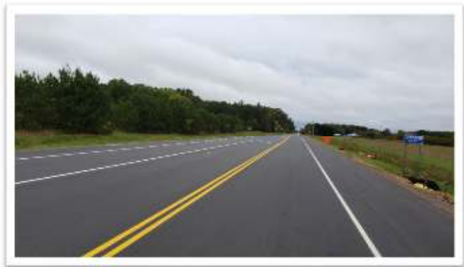
County road 78 completed
