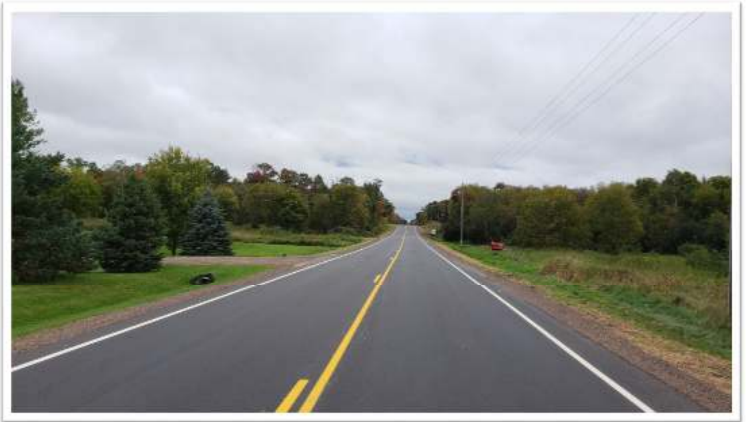
County road 78 completed
