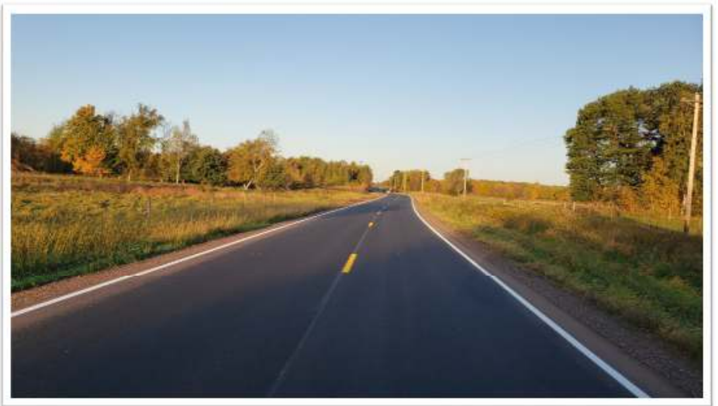
County Road 59 Completed.
