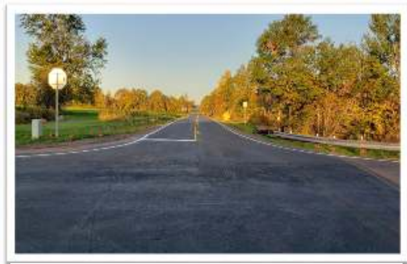
County Road 59 Completed.
