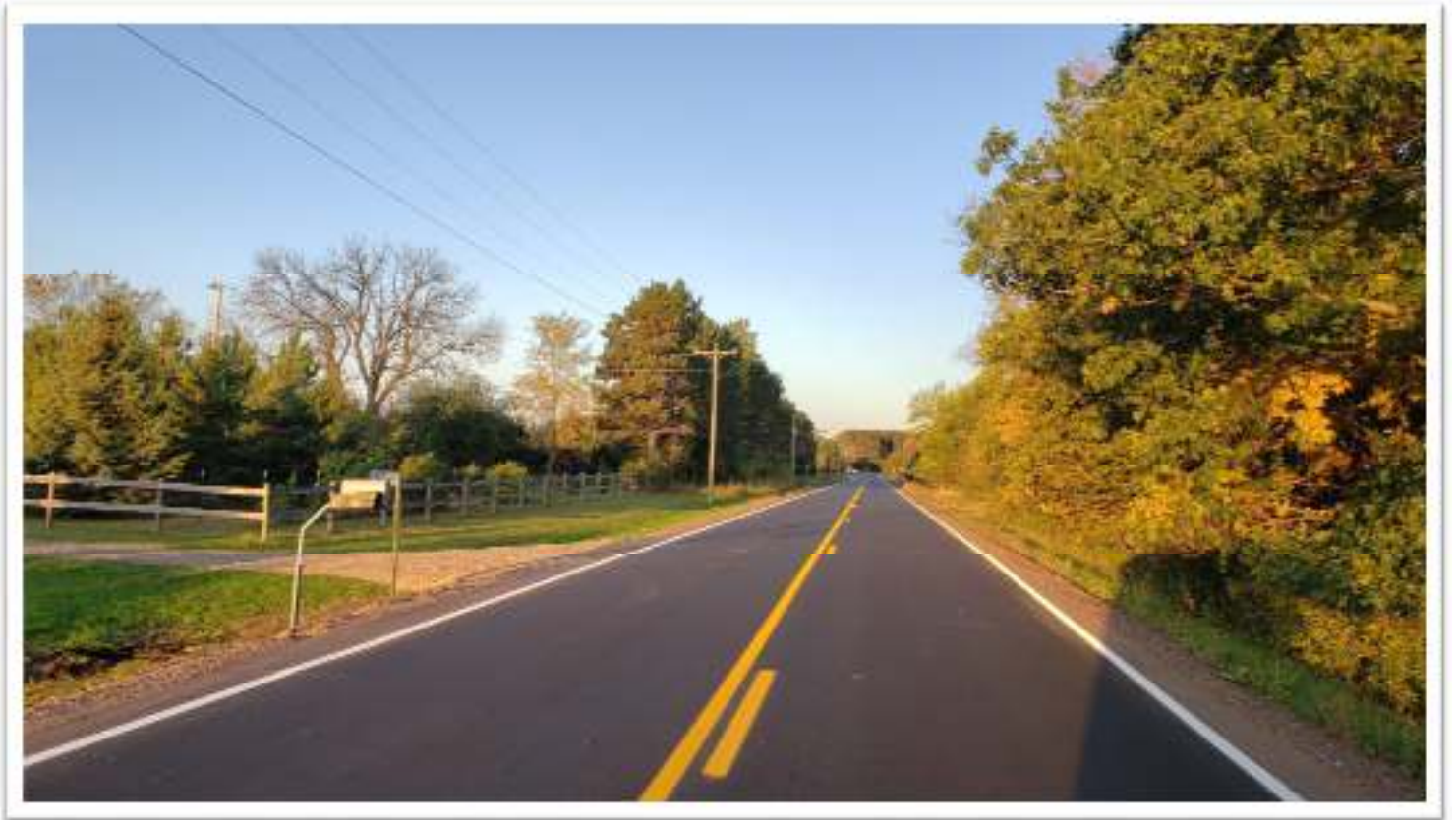
County Road 81 Completed
