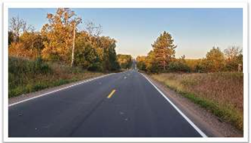
County Road 81 Completed
