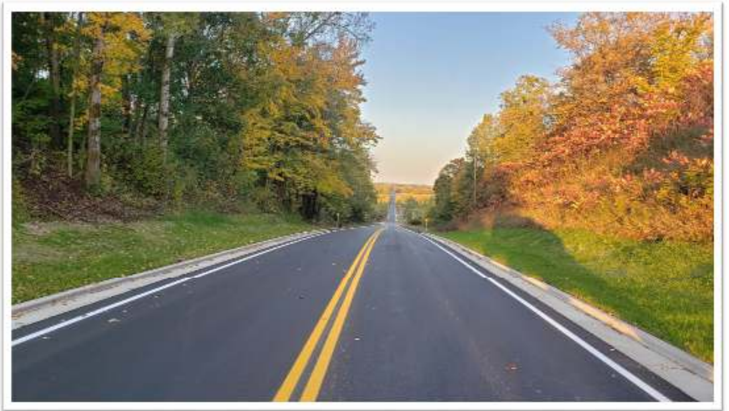
County Road 81 Completed
