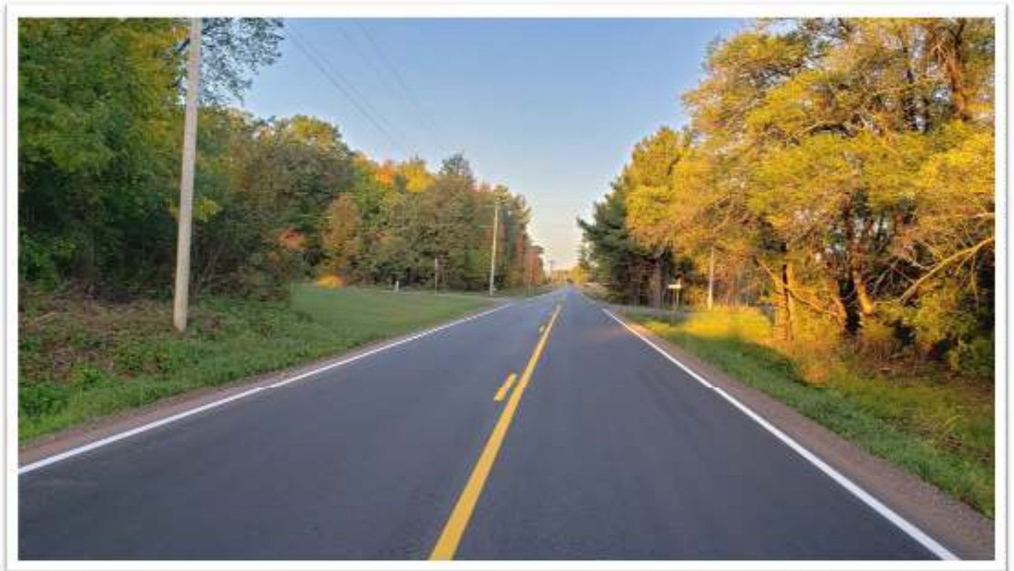
County Road 81 Completed
