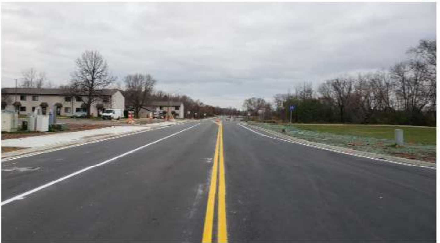
New pavement markings in place
