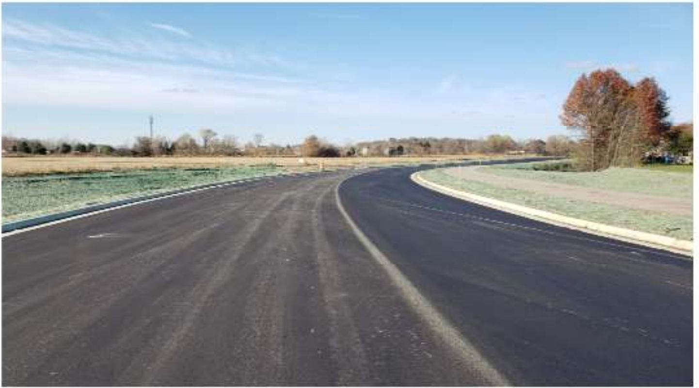
Final layer of pavement placed
