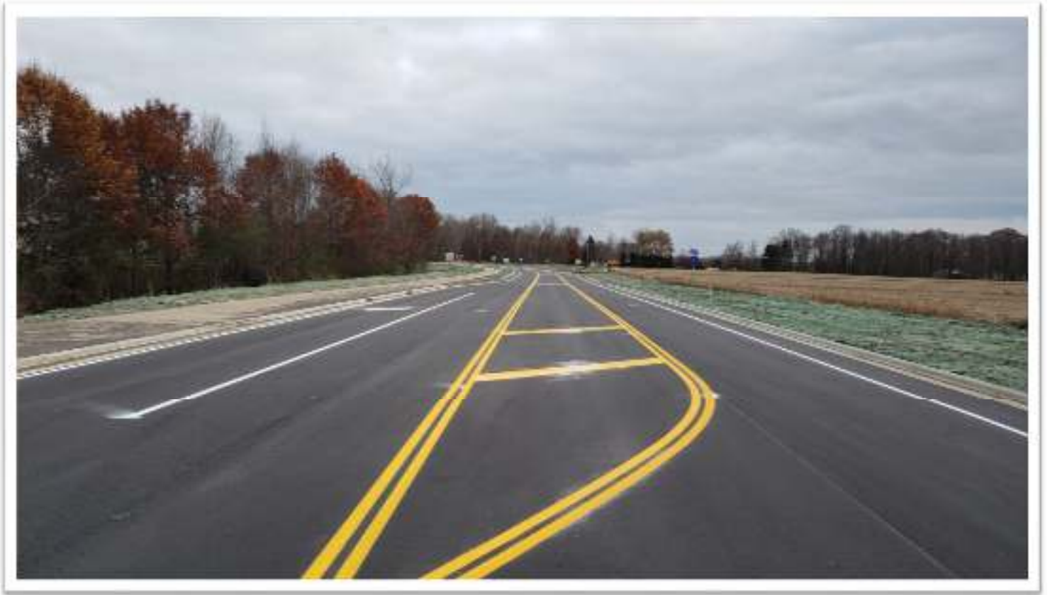
New pavement markings in place
