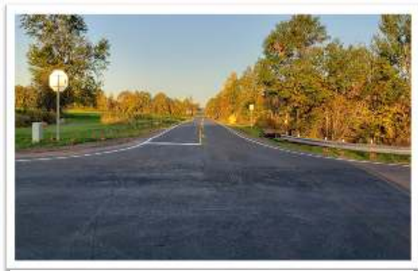
County Road 59 Completed.
