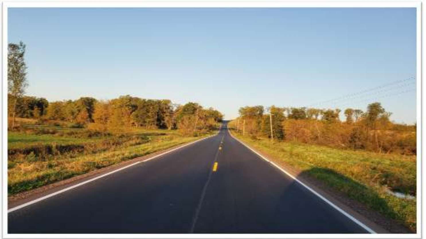
County Road 59 Completed.
