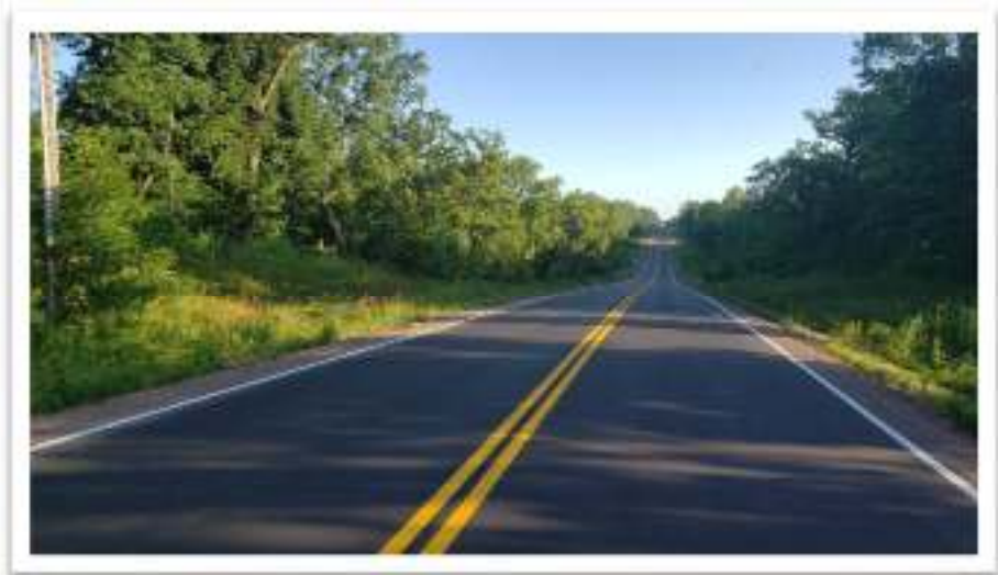
New pavement markings
