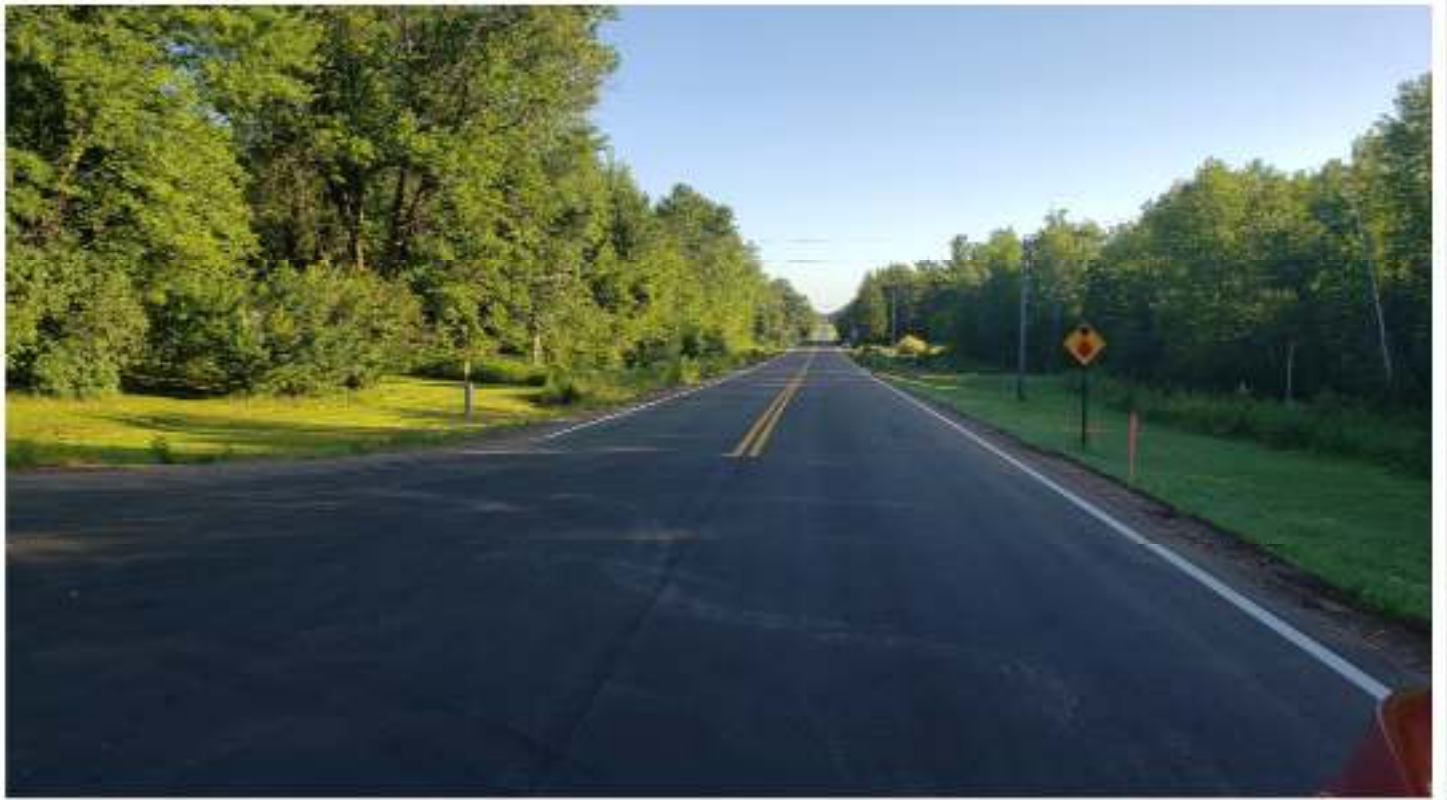
New pavement markings
