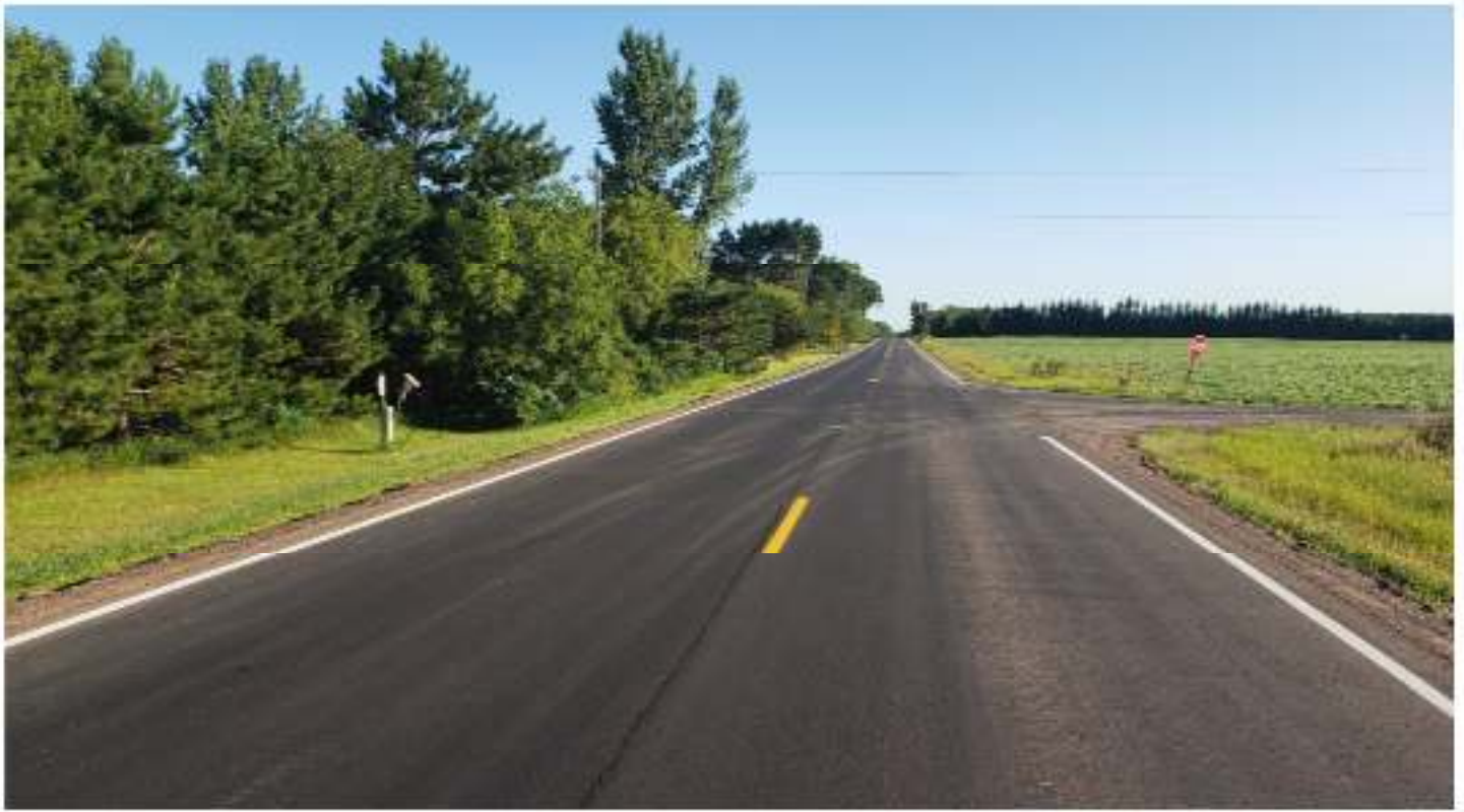
New pavement markings
