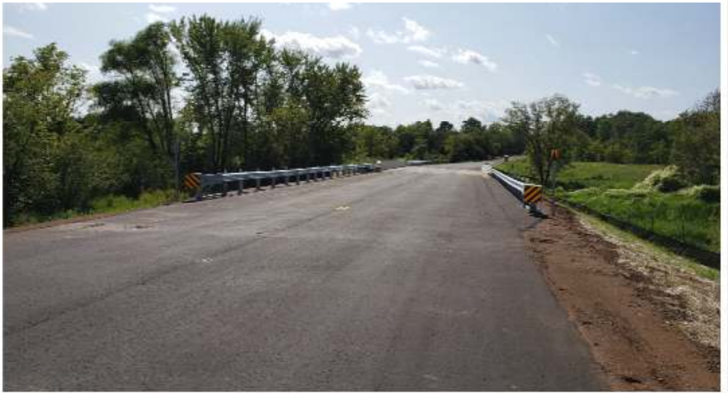
New guard railings
