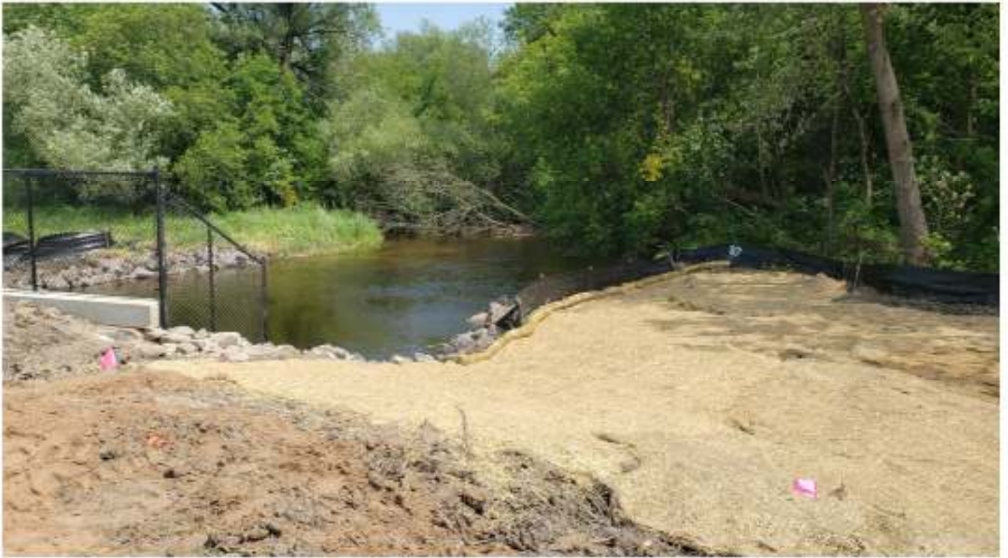
Erosion control and turf establishment
