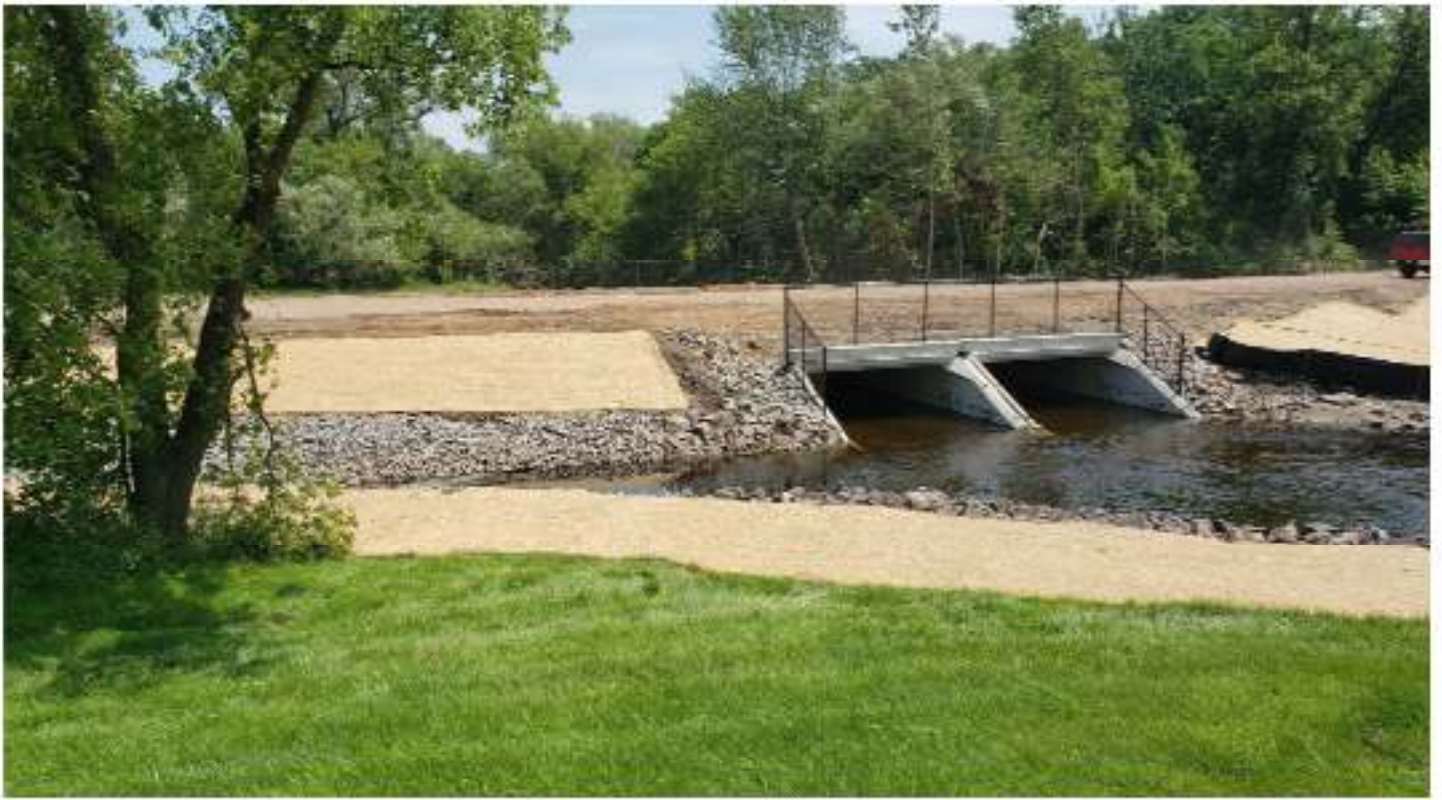
Erosion control and turf establishment on West banks
