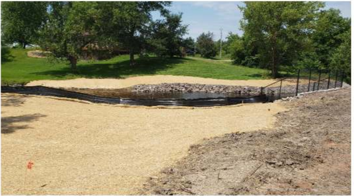
Erosion control and turf establishment
