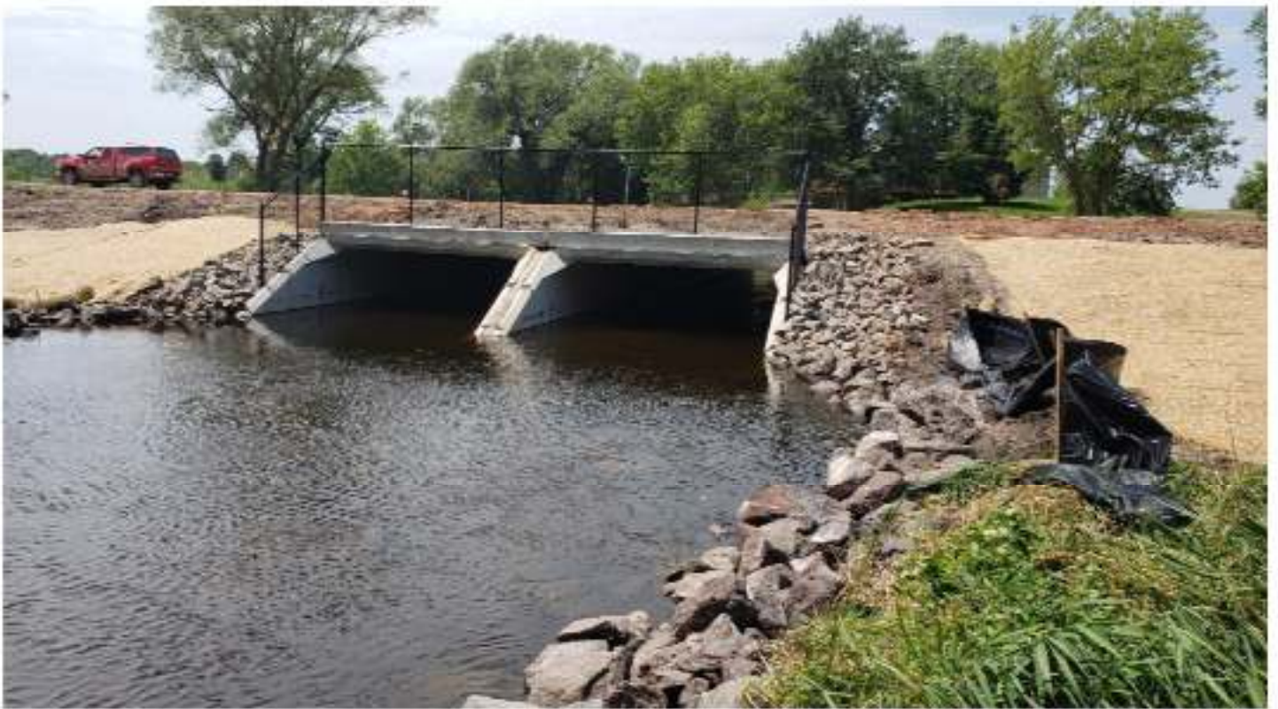
East bank safety fencing and rip rap
