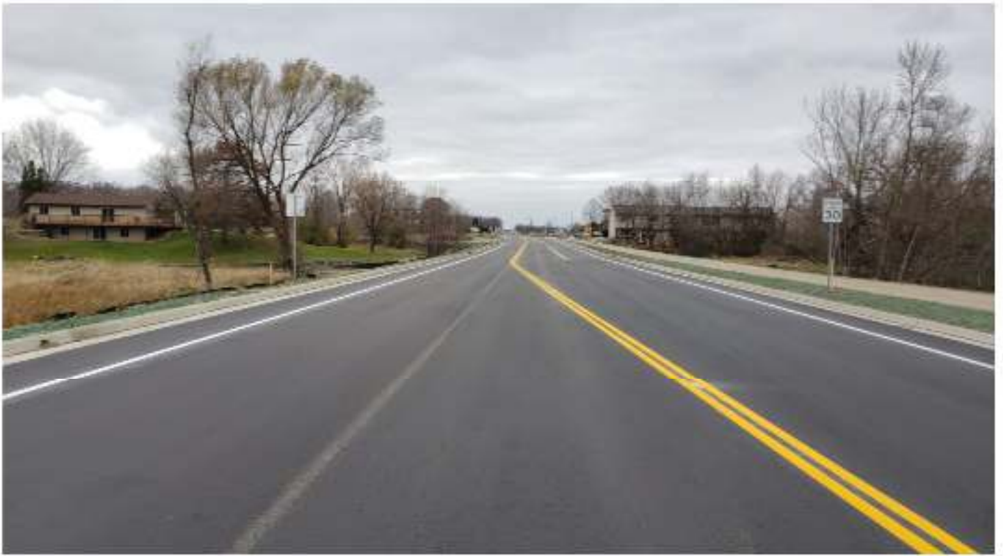
New pavement markings in place
