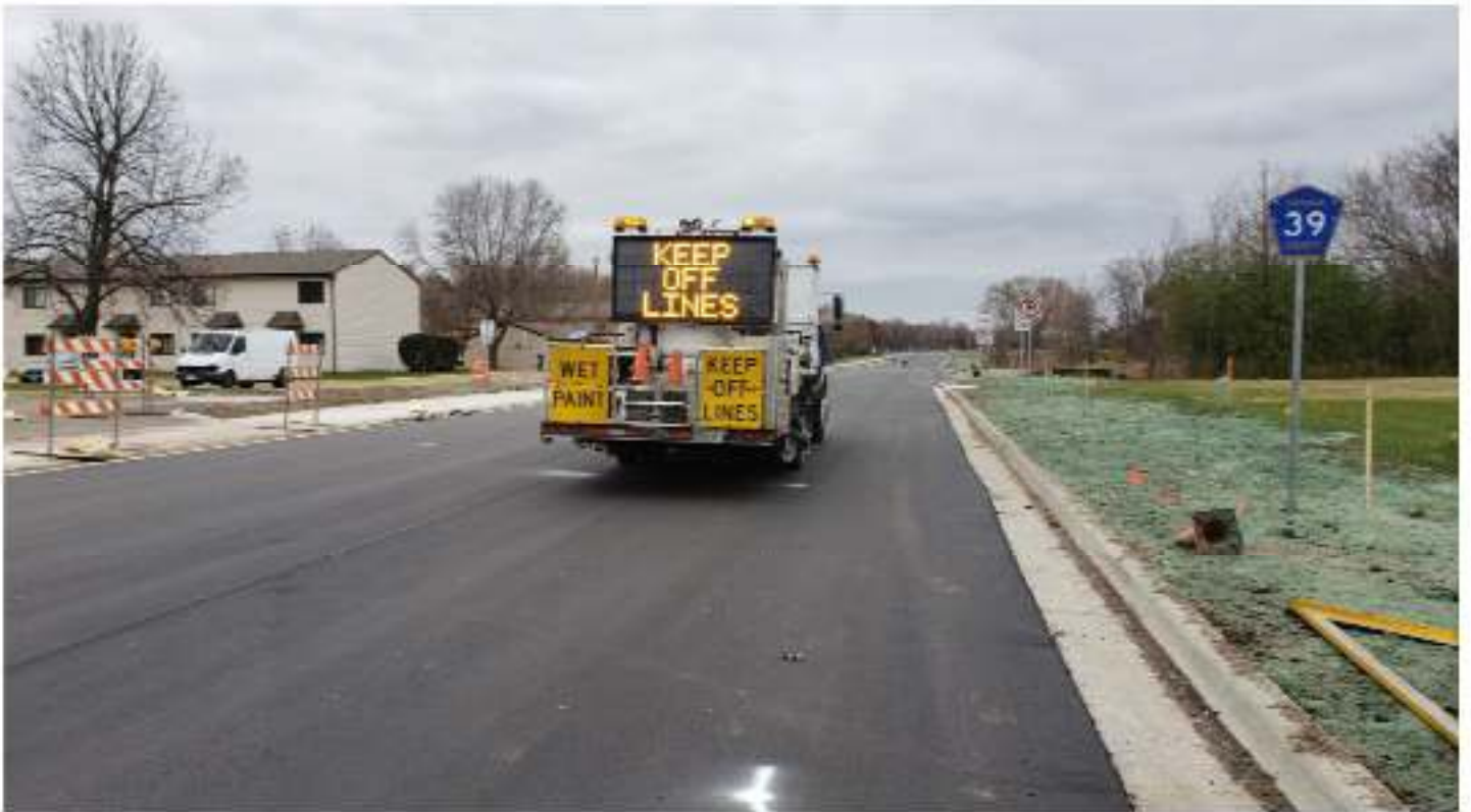
Prepping to place new pavement markings
