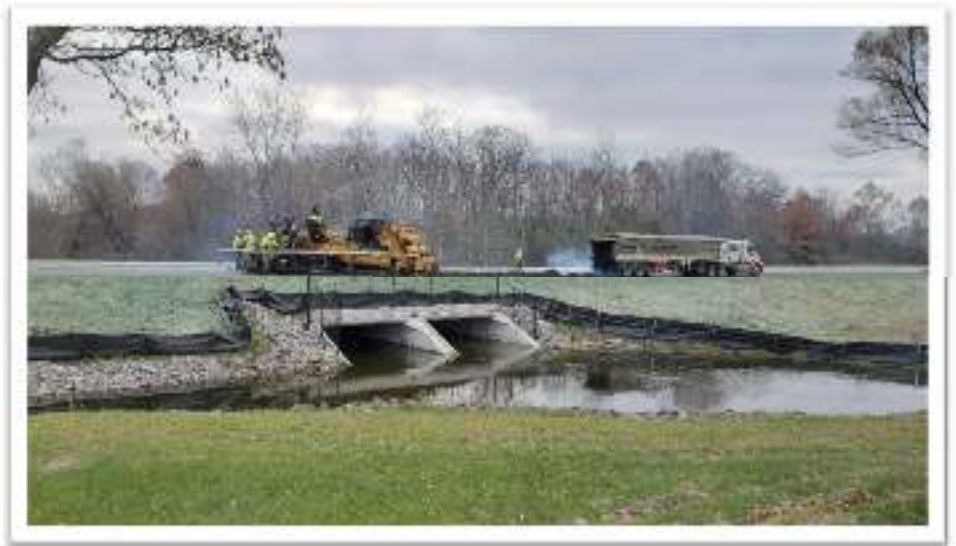
Final Layer of pavement being placed over Rush Creek
