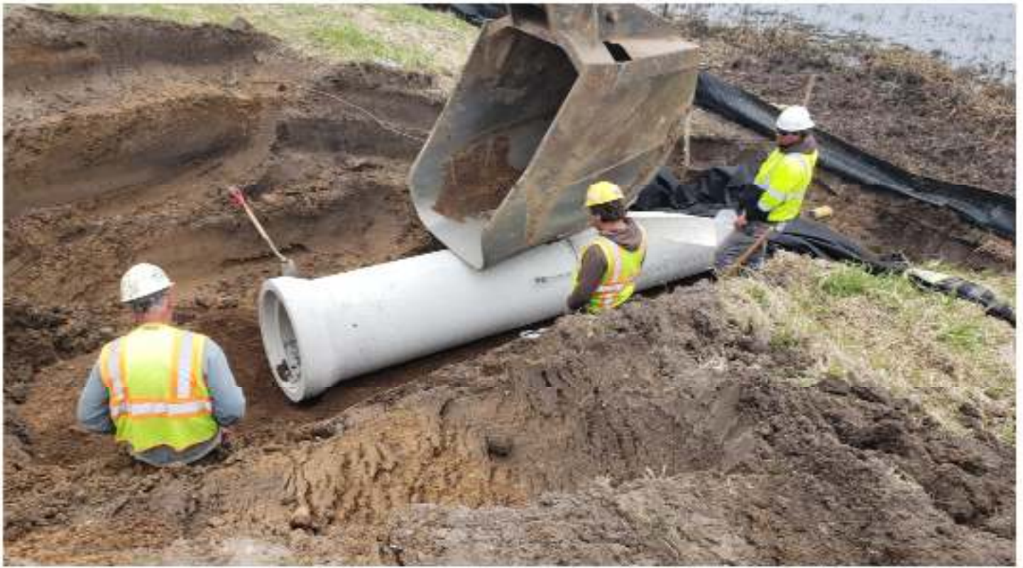
Installing New Storm Sewer
