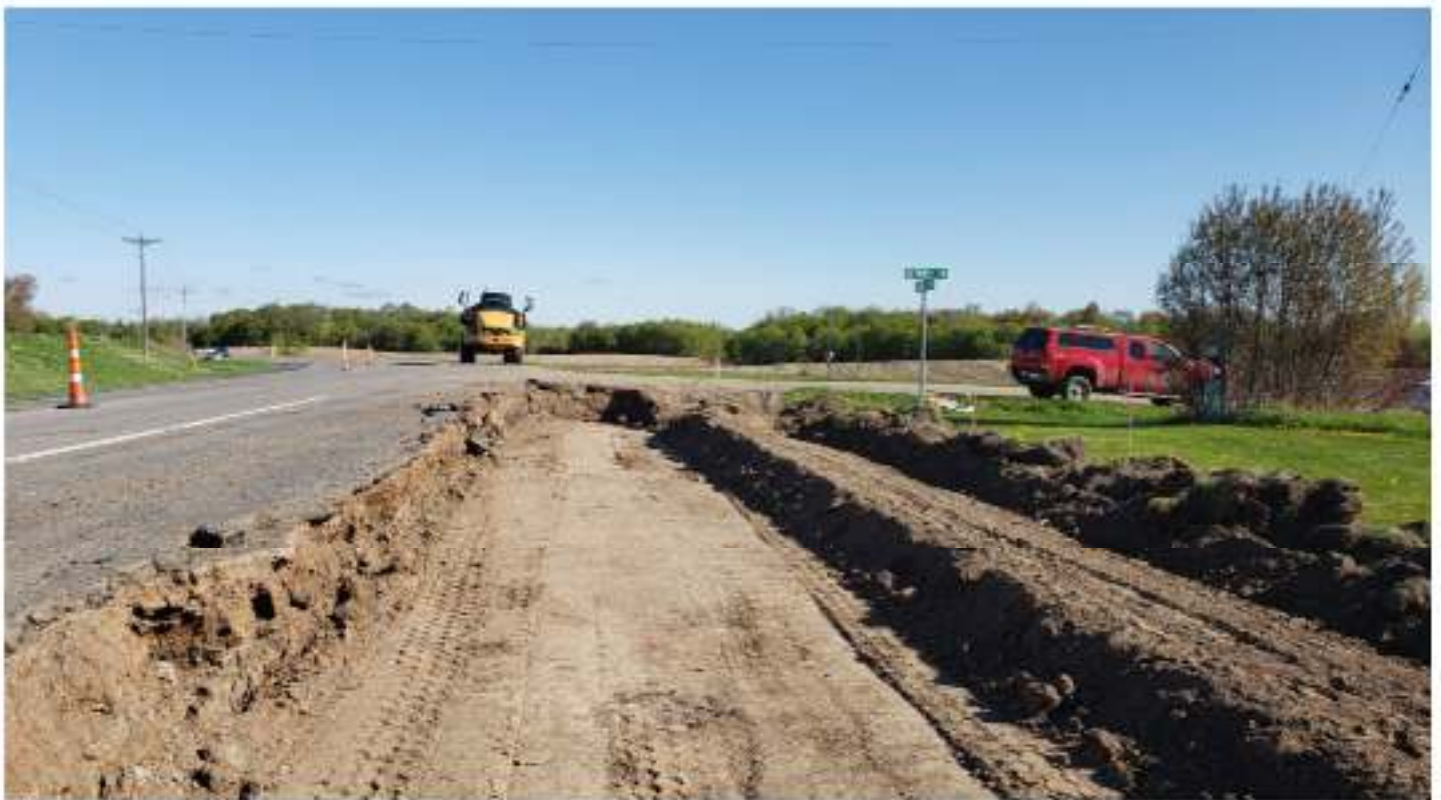
New Right Turn Lane Being Installed.
