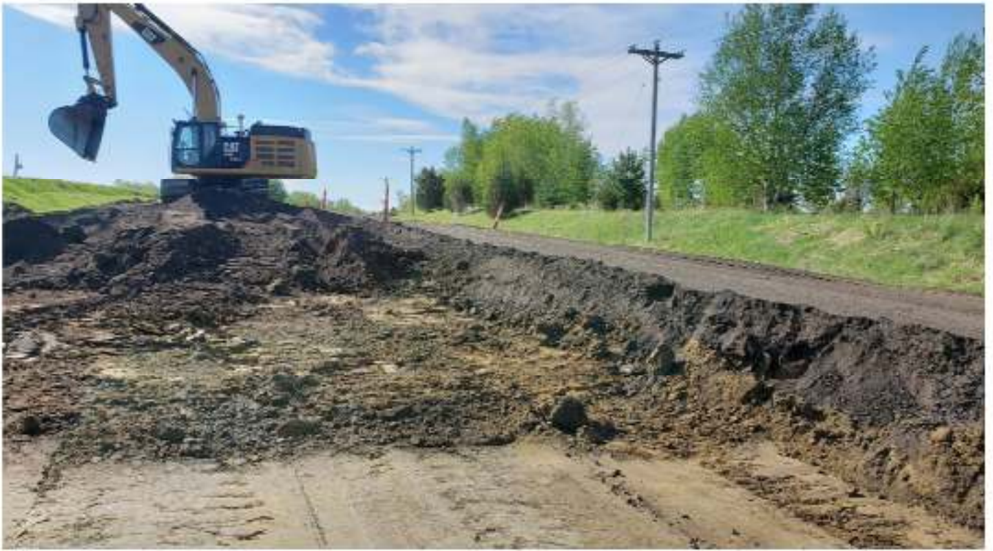
Soil Correction Area
