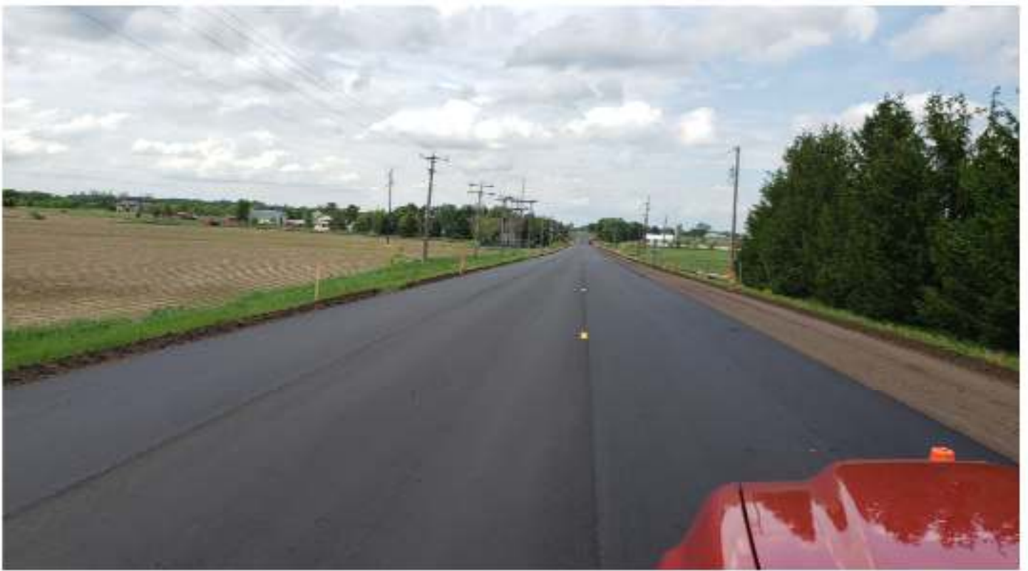
Base Course Of New Pavement
