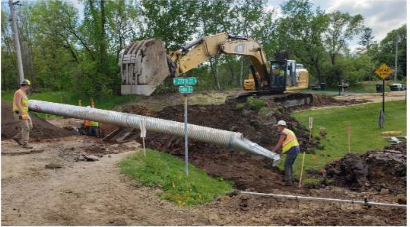
New Culvert Being Installed
