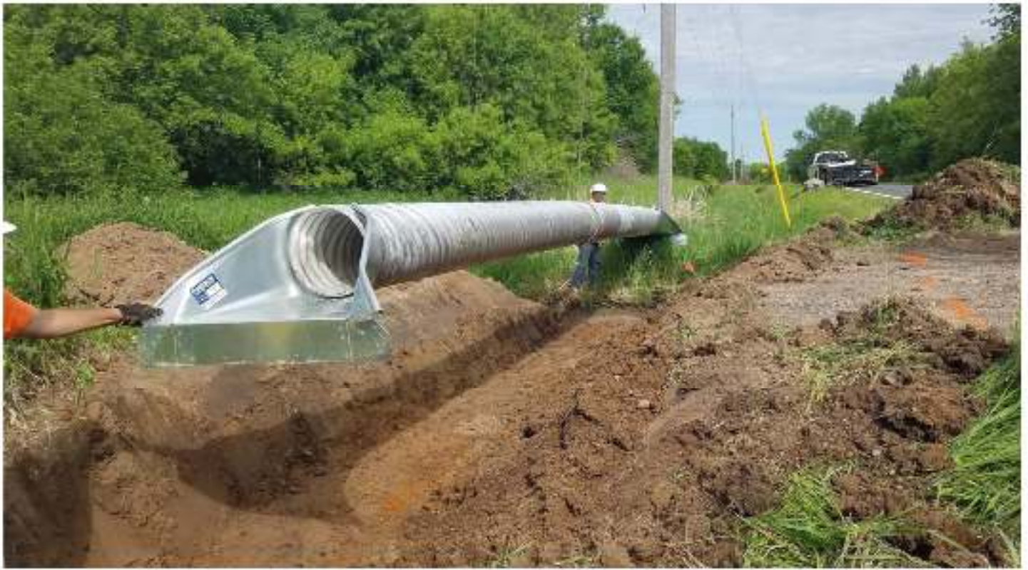
New Drive Way Culvert Being Installed
