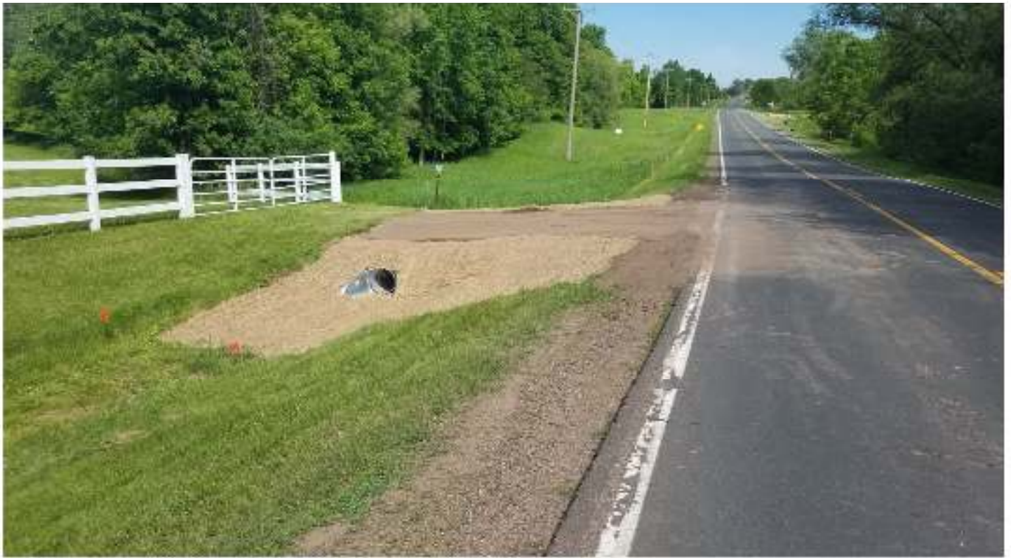
New Drive Way Culvert Installed
