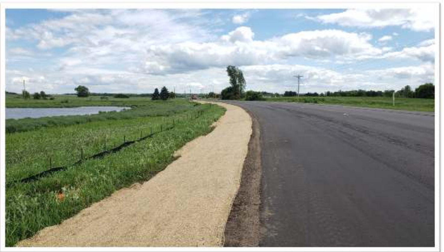
Installed Seed and Straw Blanket
