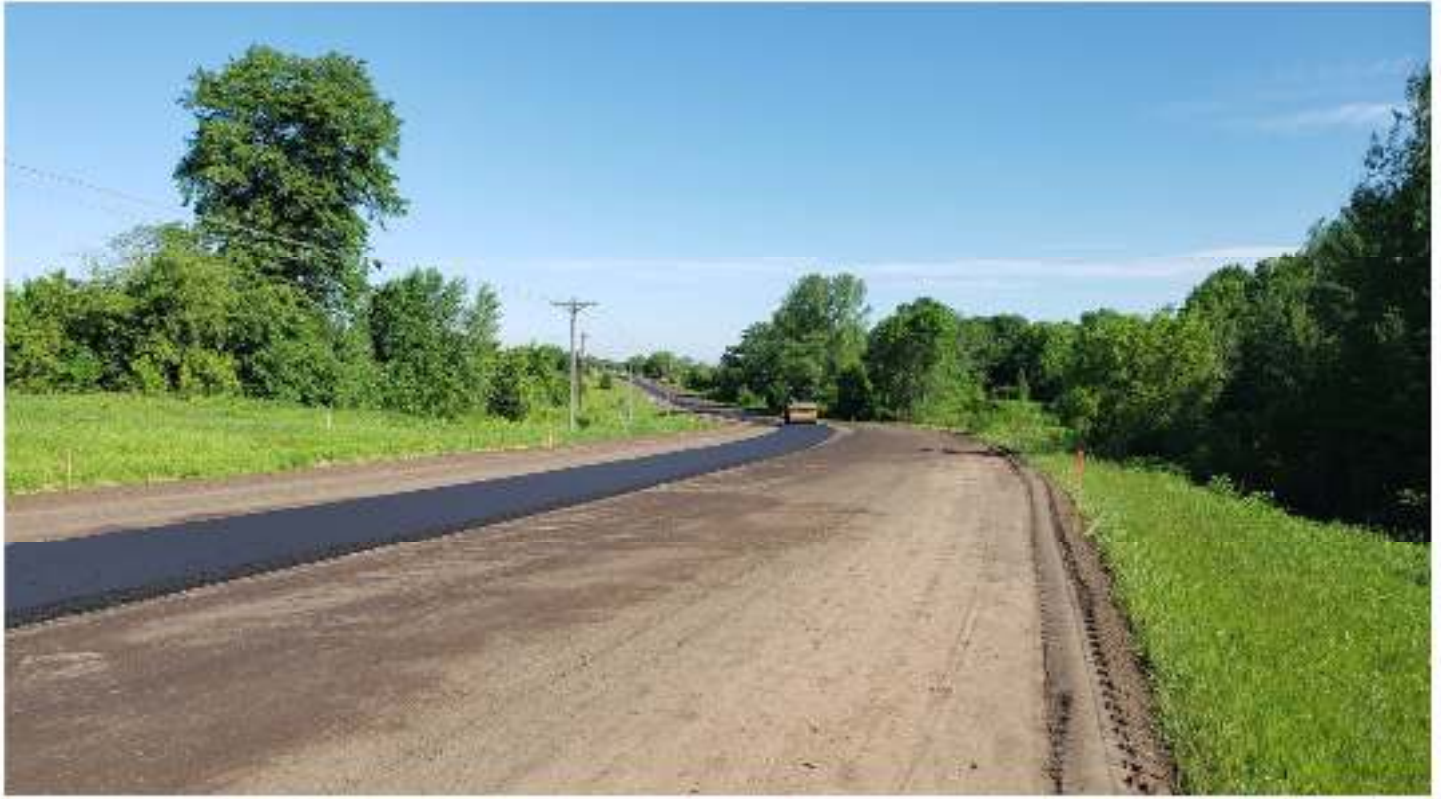
First Layer of Pavement
