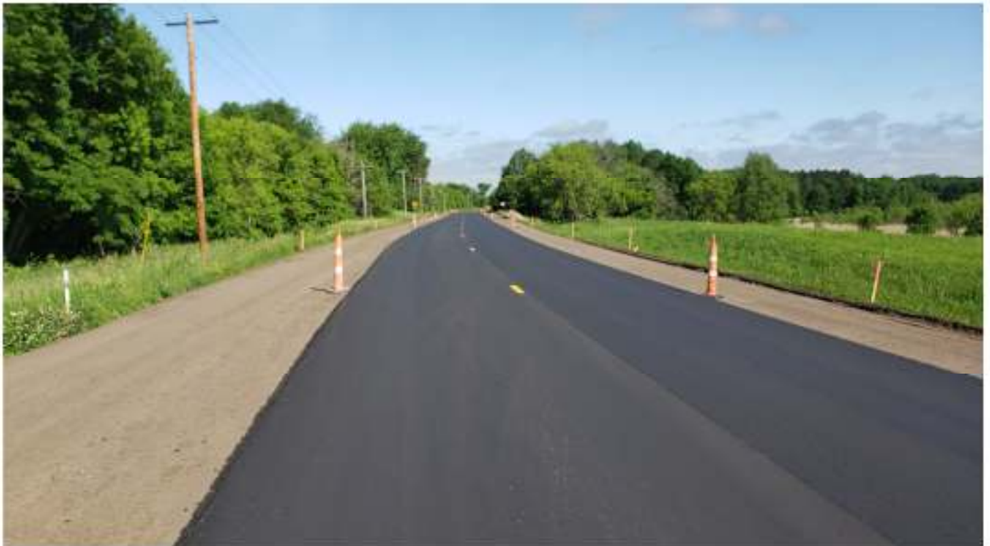
First Layer of Pavement
