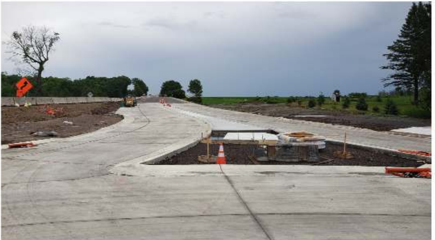
New Concrete Pavement
