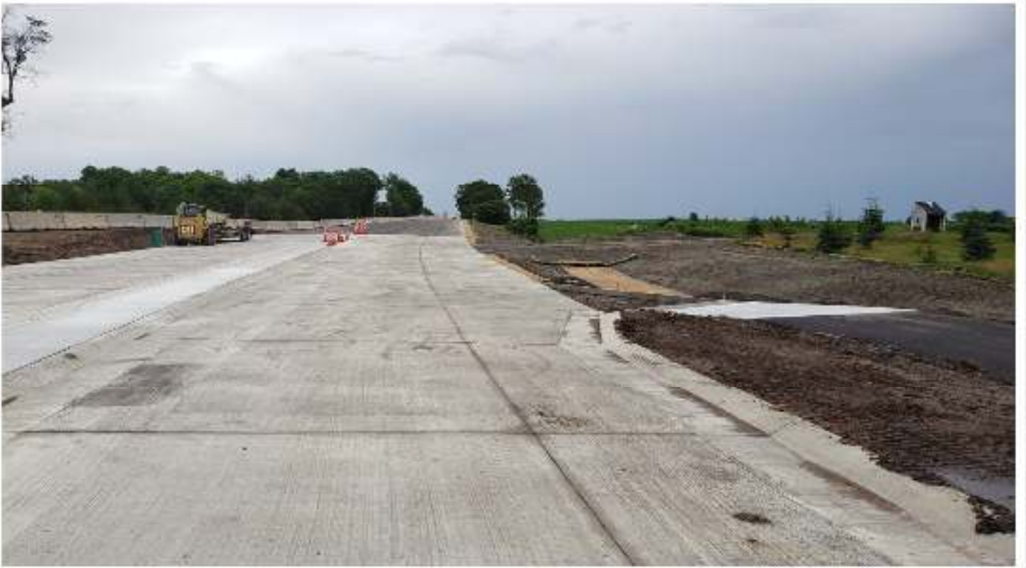
New Concrete Pavement
