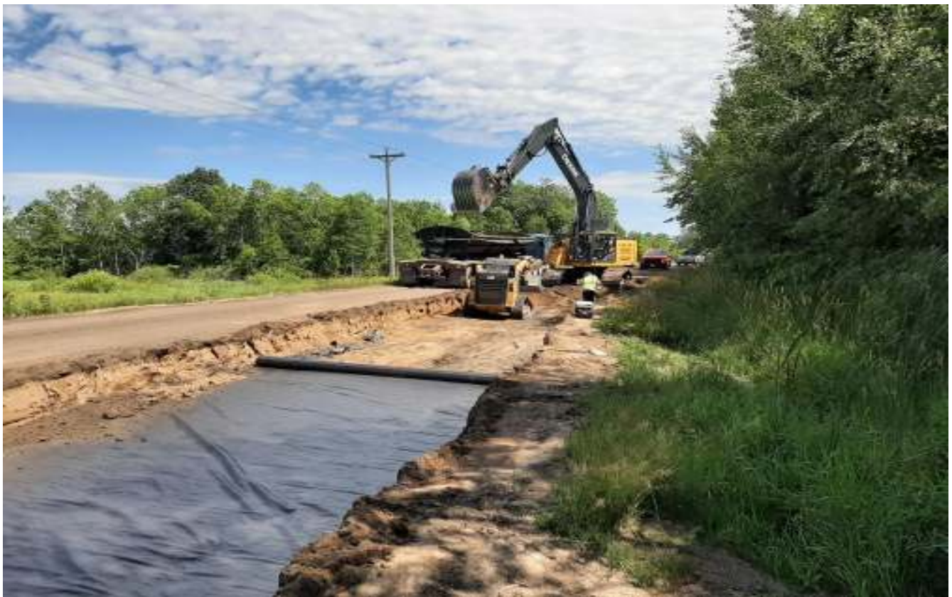
Sub cutting Road
