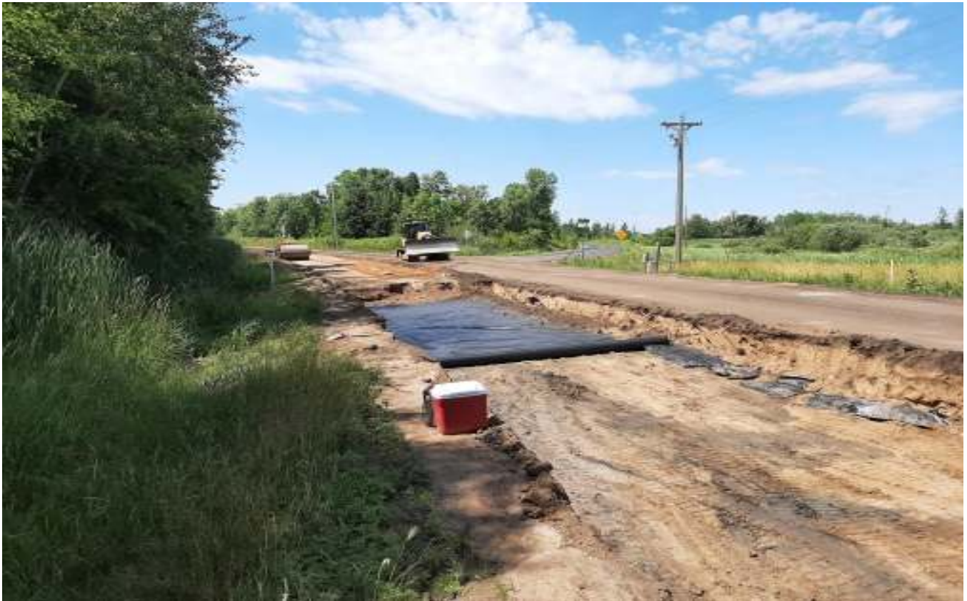
Sub cutting Road
