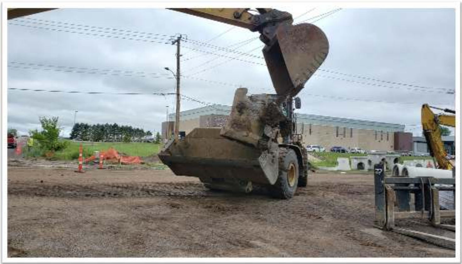
Removing Old Storm Sewer
