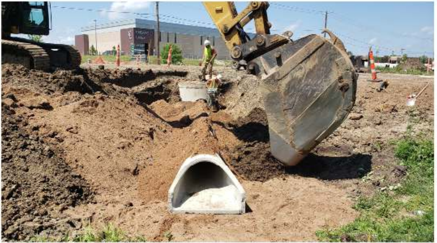
New Storm Sewer Pipe
