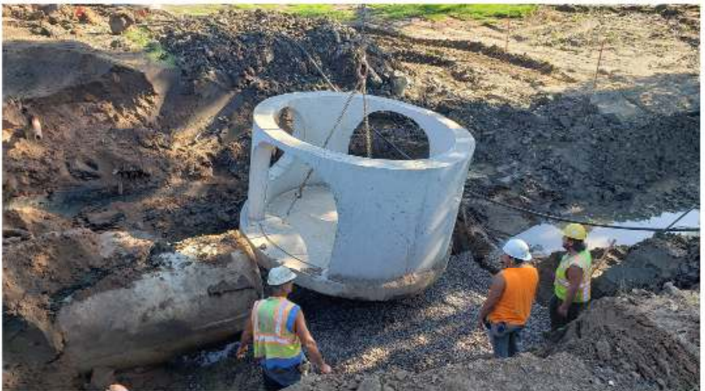
New Storm Sewer Pipe
