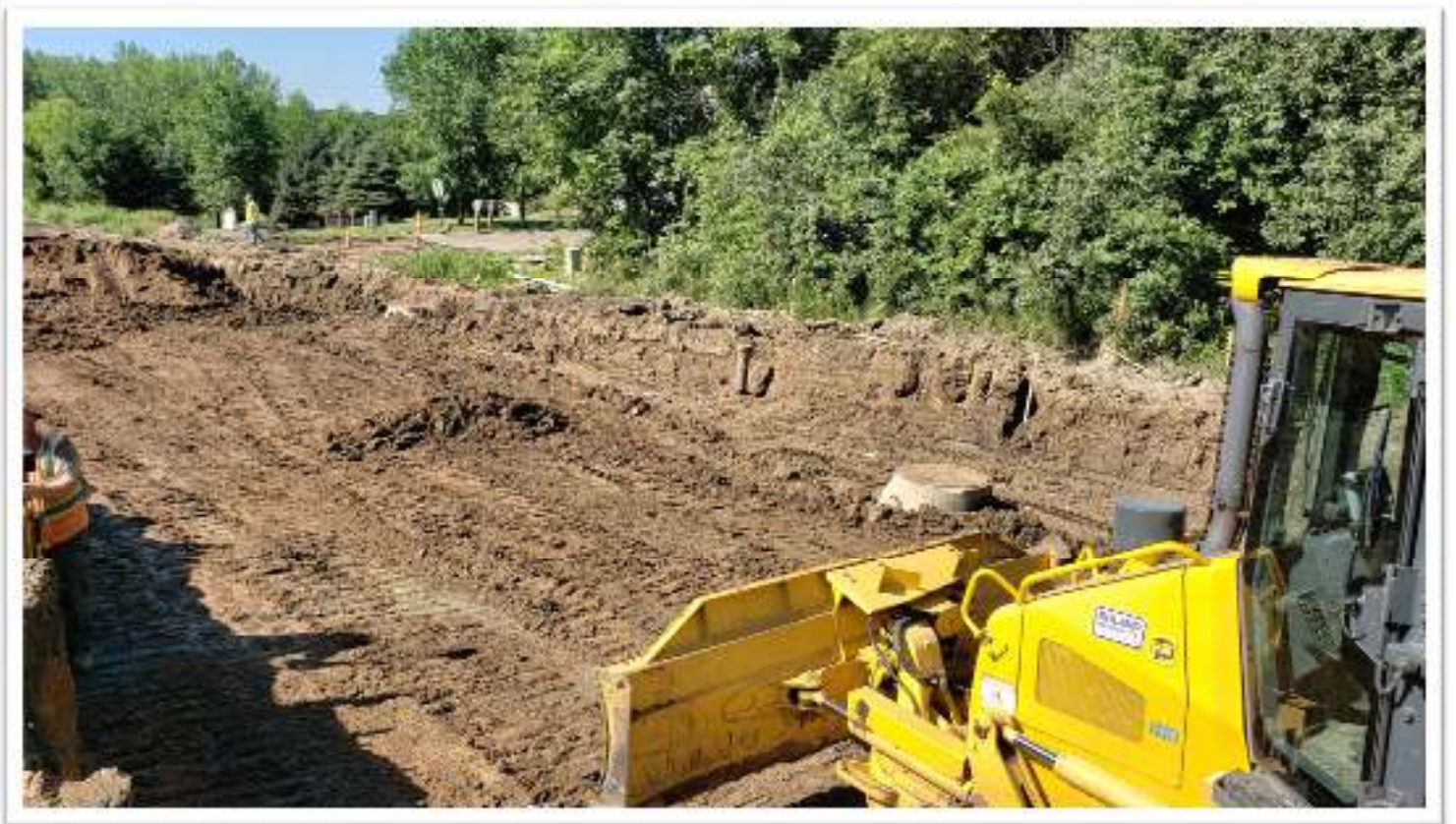
Sub cutting road
