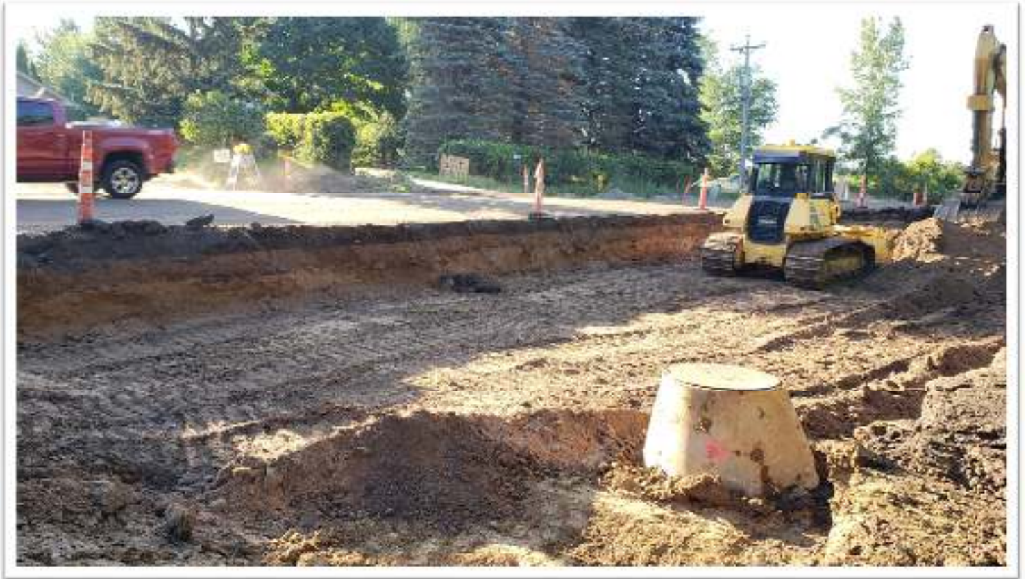
Sub cutting road
