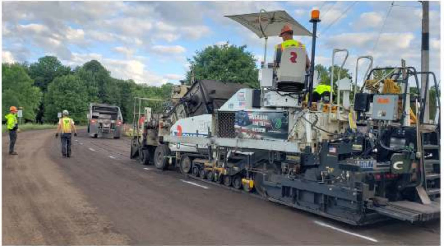
New Pavement Being Placed
