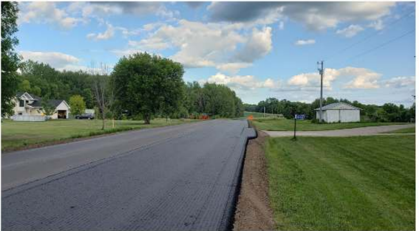
New Pavement Being Placed
