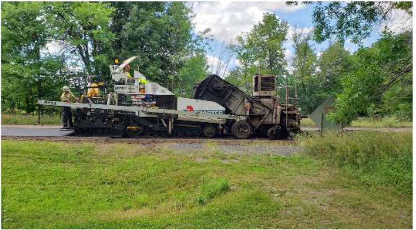
Road Paver At Work
