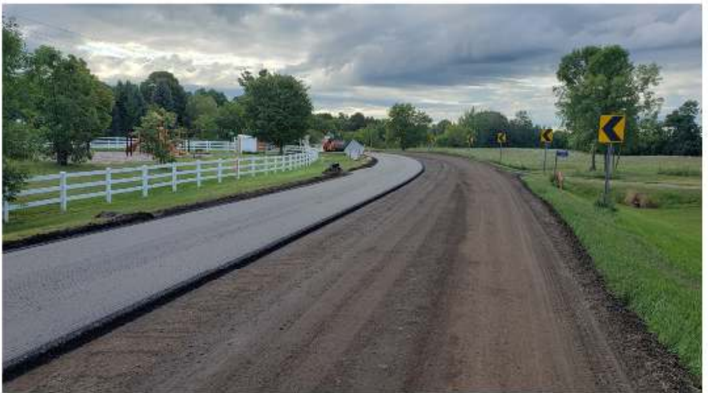
New Pavement Being Placed
