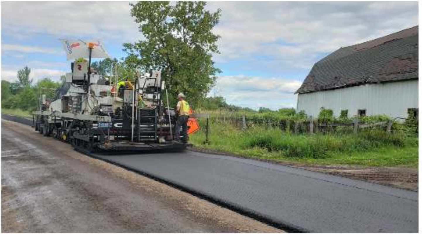
New Pavement Being Placed
