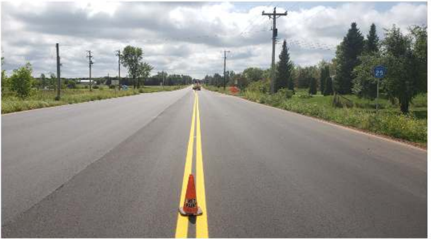
New Pavement Markings
