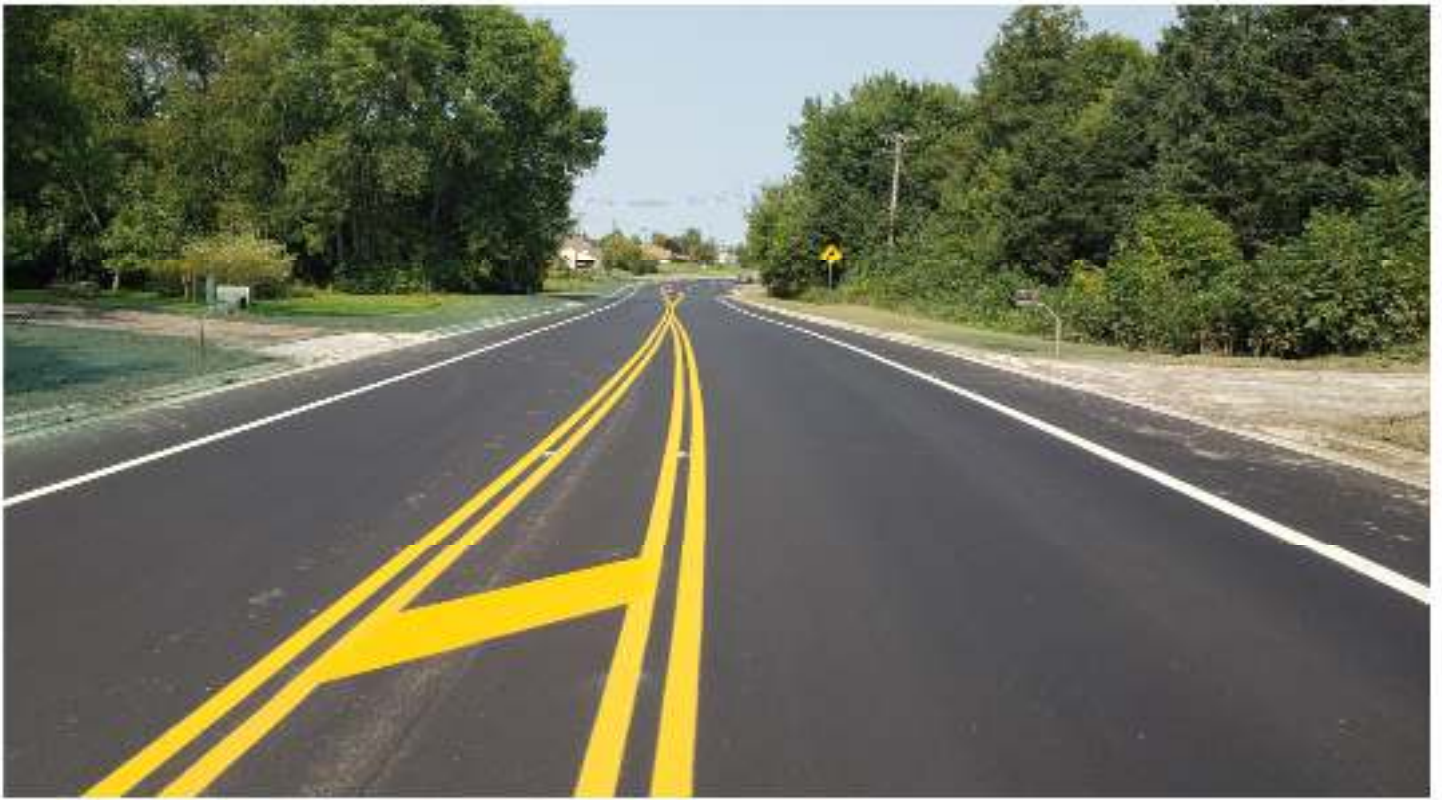
New Pavement Markings
