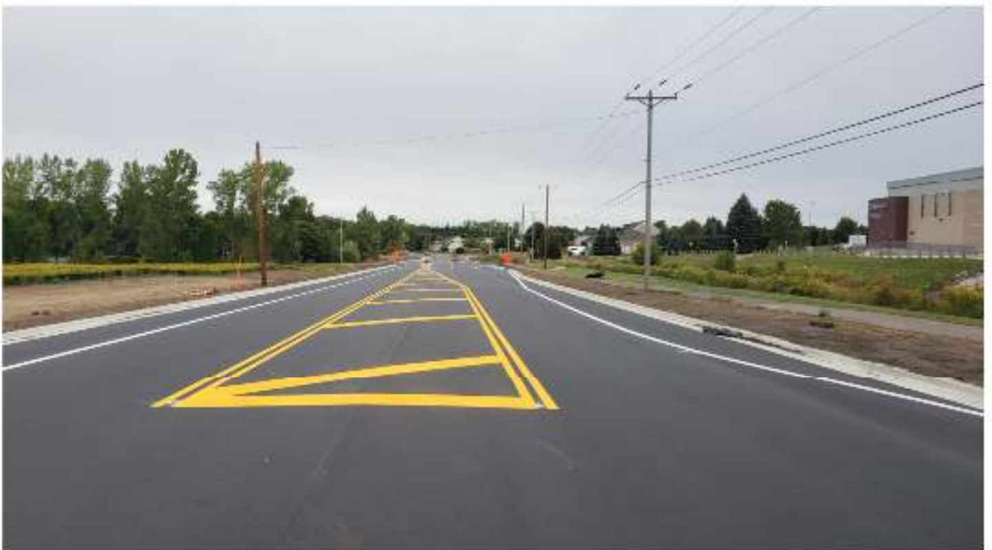
New Pavement Markings
