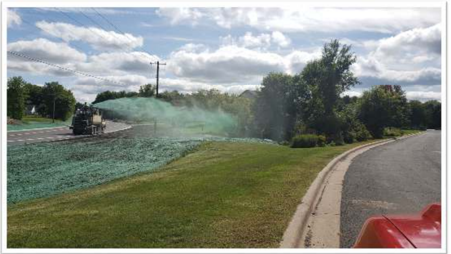
Hydro-mulch and Seeding
