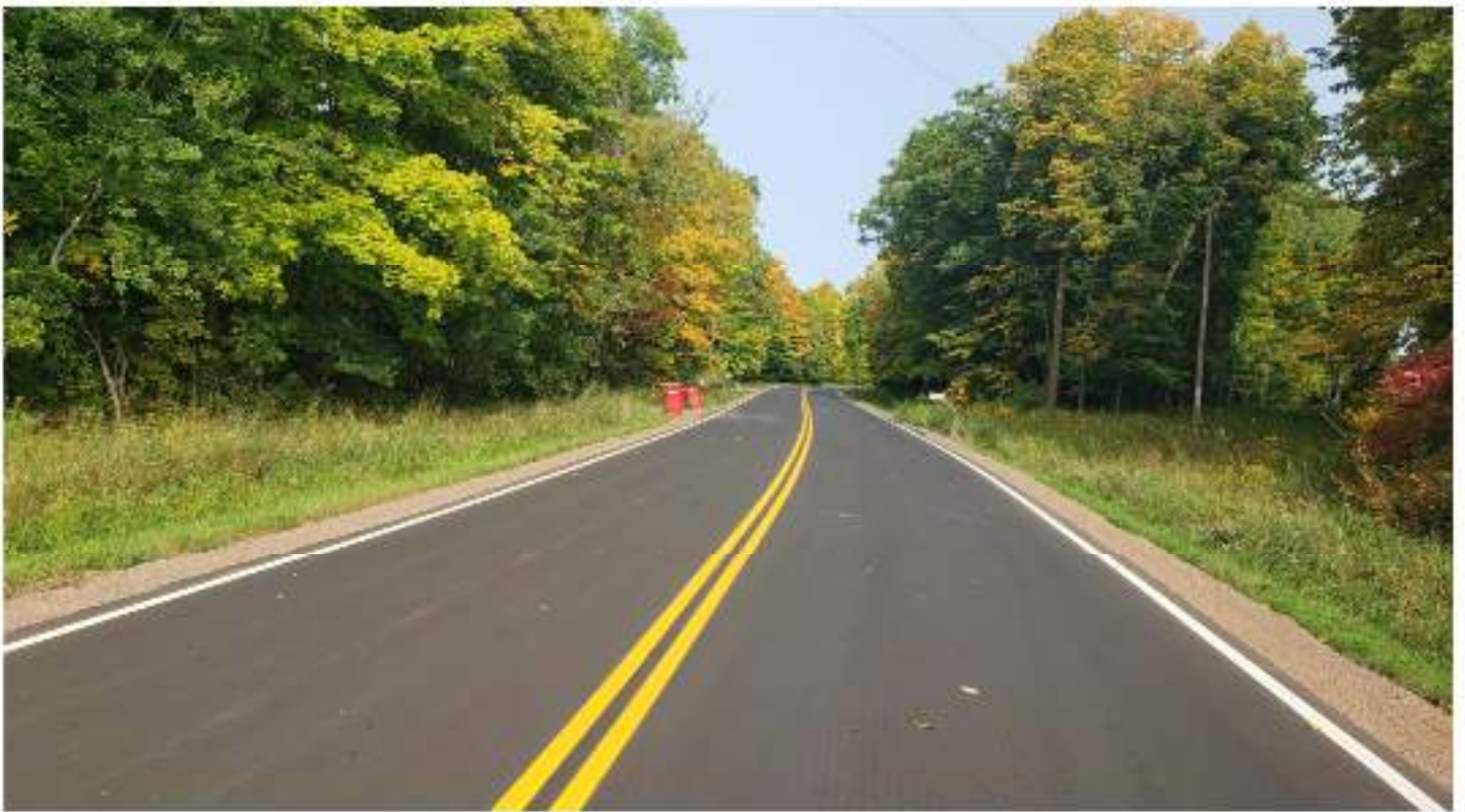
New pavement and markings
