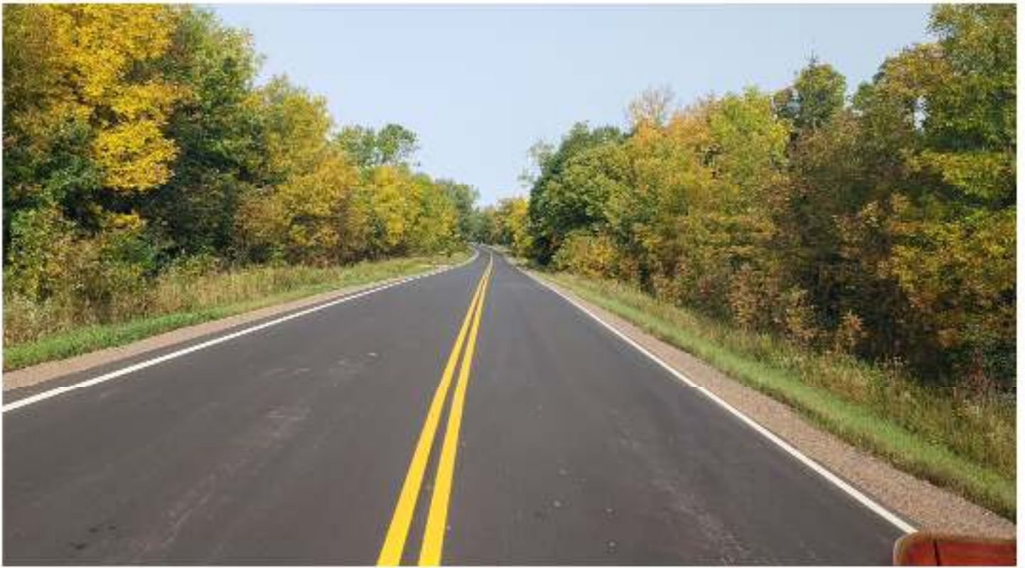
New pavement and markings
