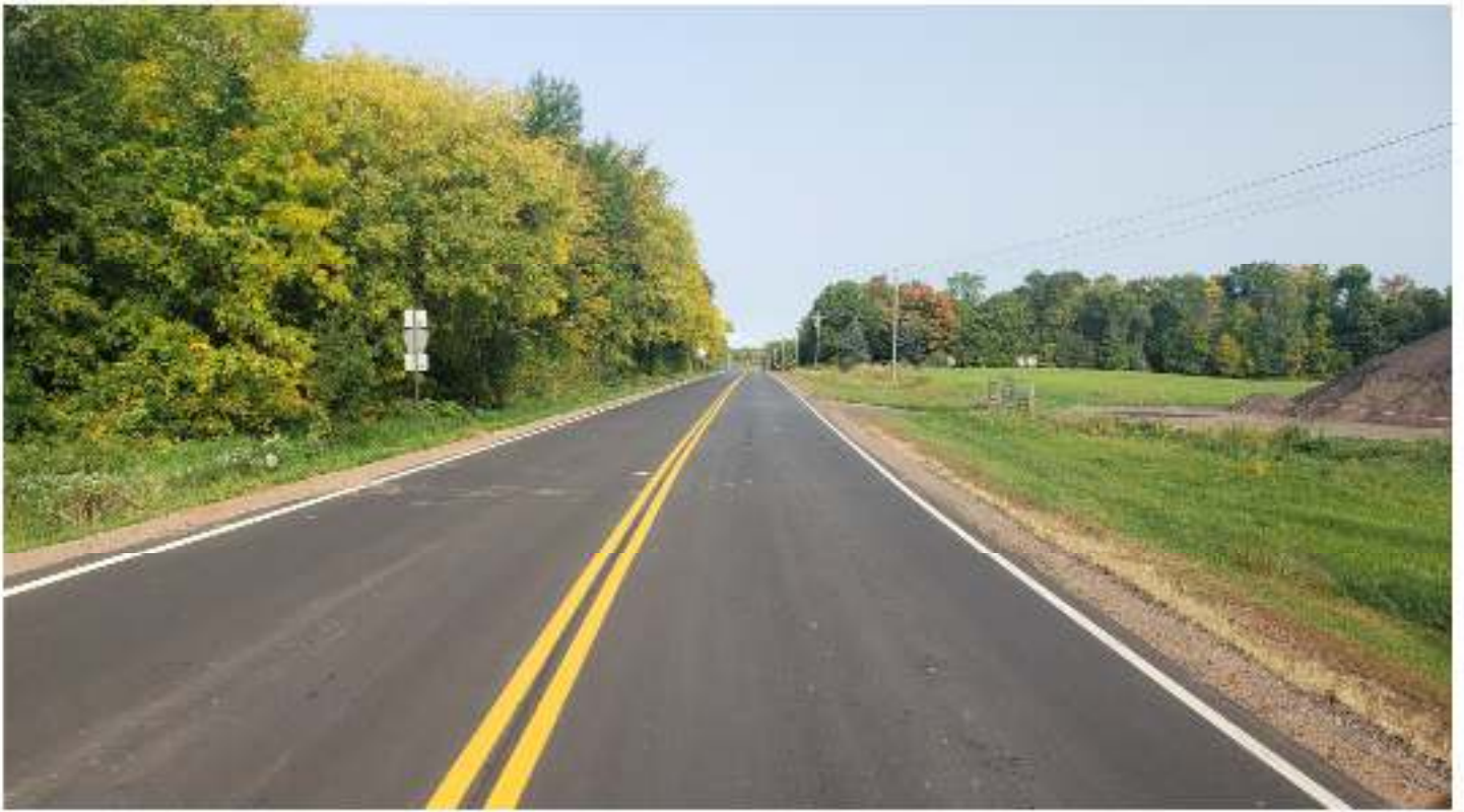
New pavement and markings
