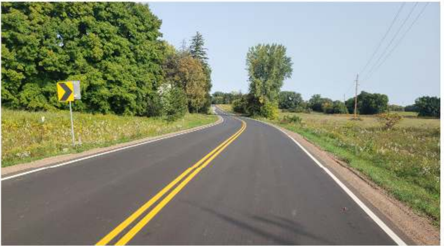
New pavement and markings
