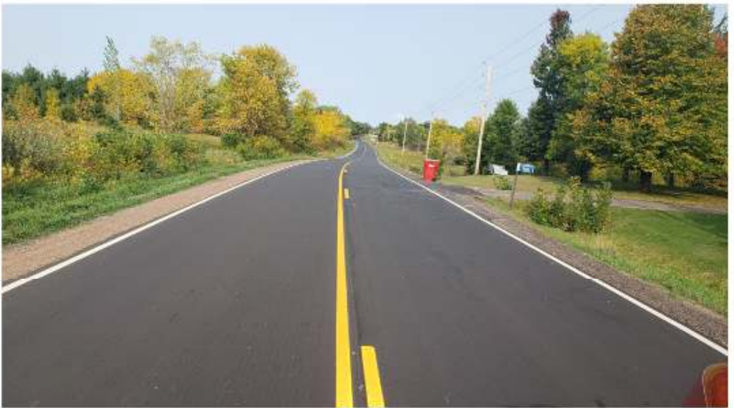
New pavement and markings
