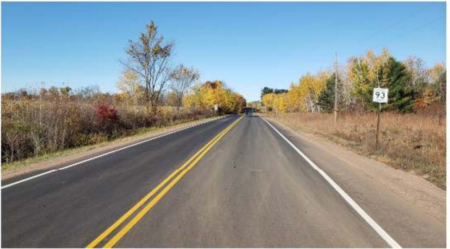
New Pavement Striping
