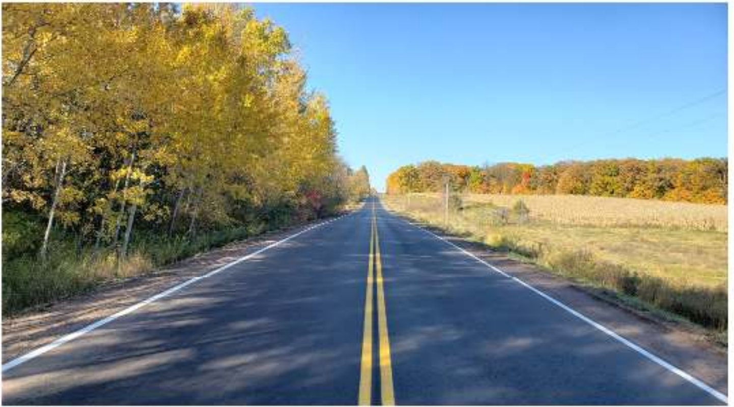
New Pavement Striping
