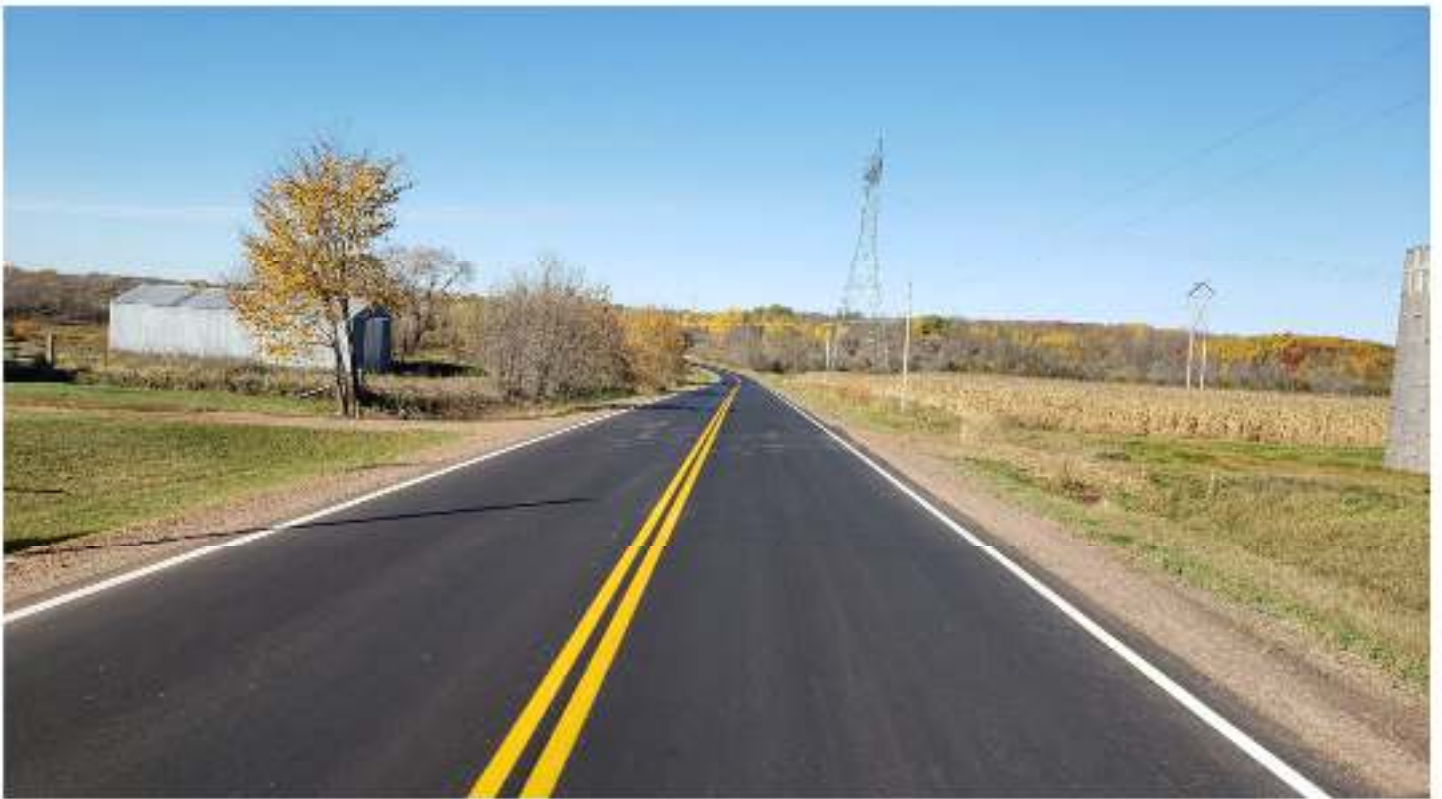
New Pavement Striping
