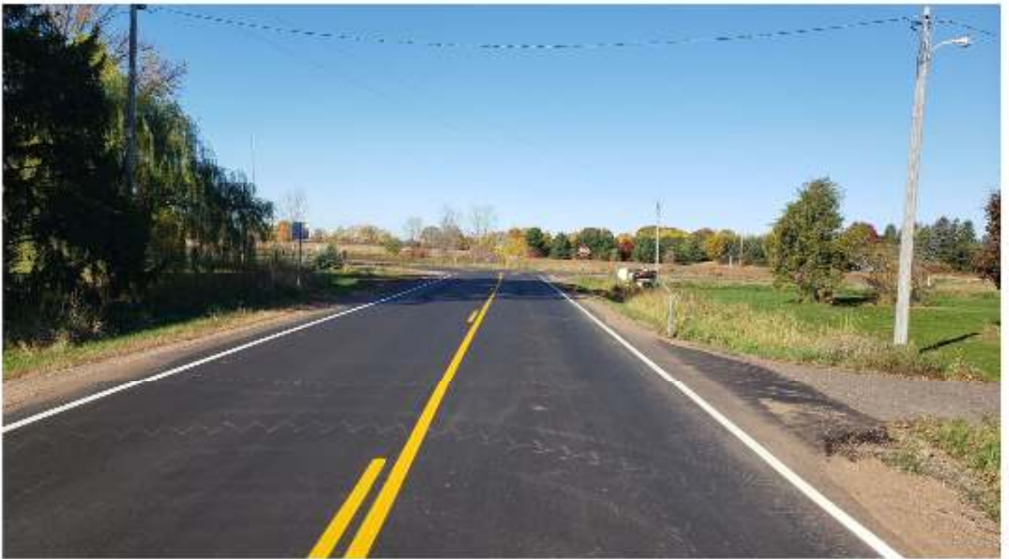
New Pavement Striping
