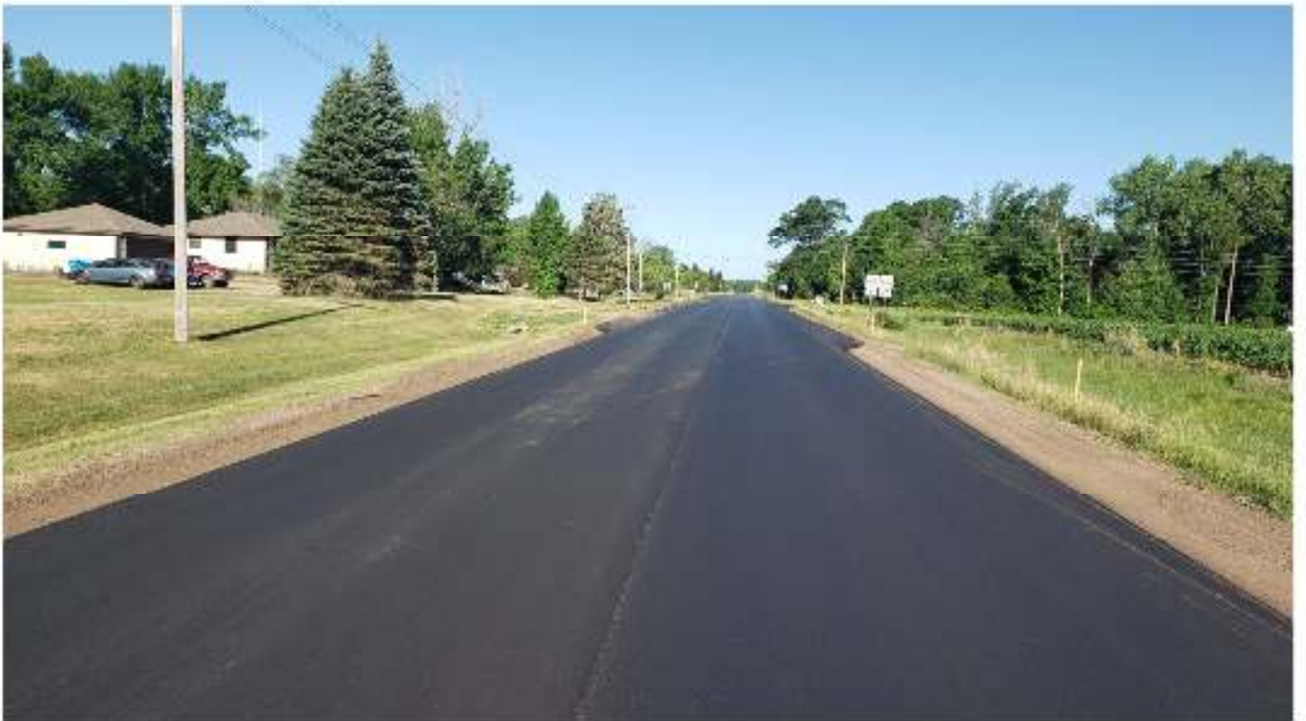
Final Course of New Pavement on CR 65
