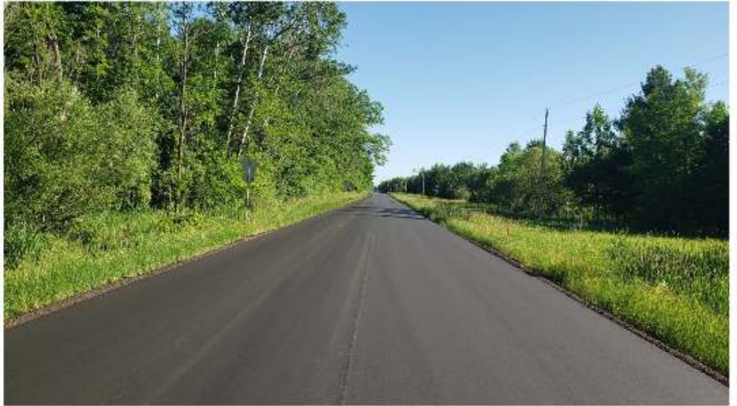
Final Course of New Pavement on CR 65
