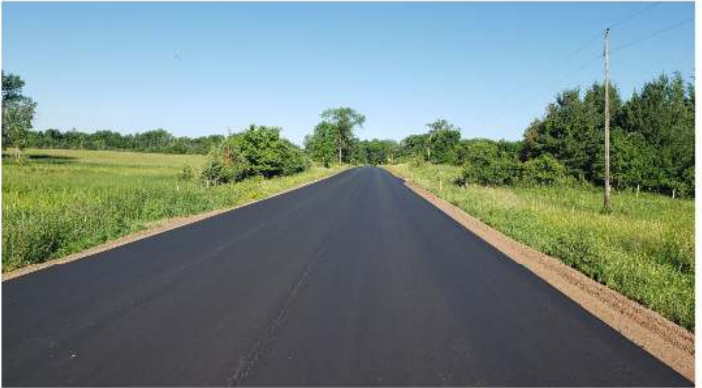
Final Course of New Pavement on CR 65
