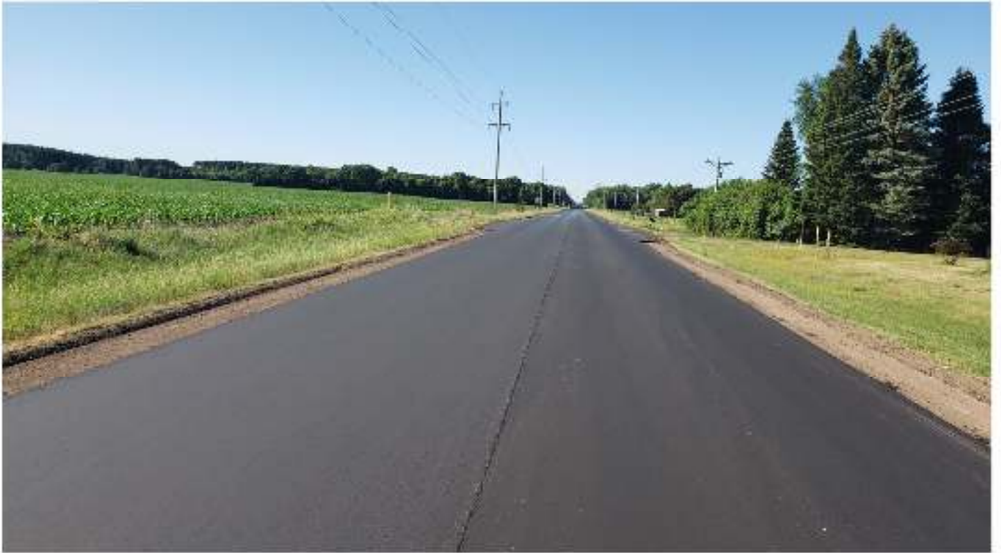
Final Course of New Pavement on CR 65
