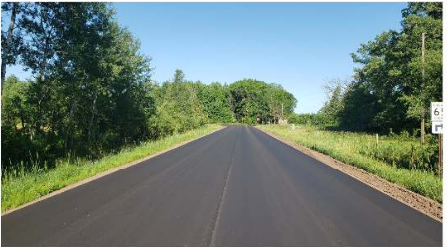
Final Course of New Pavement on CR 65
