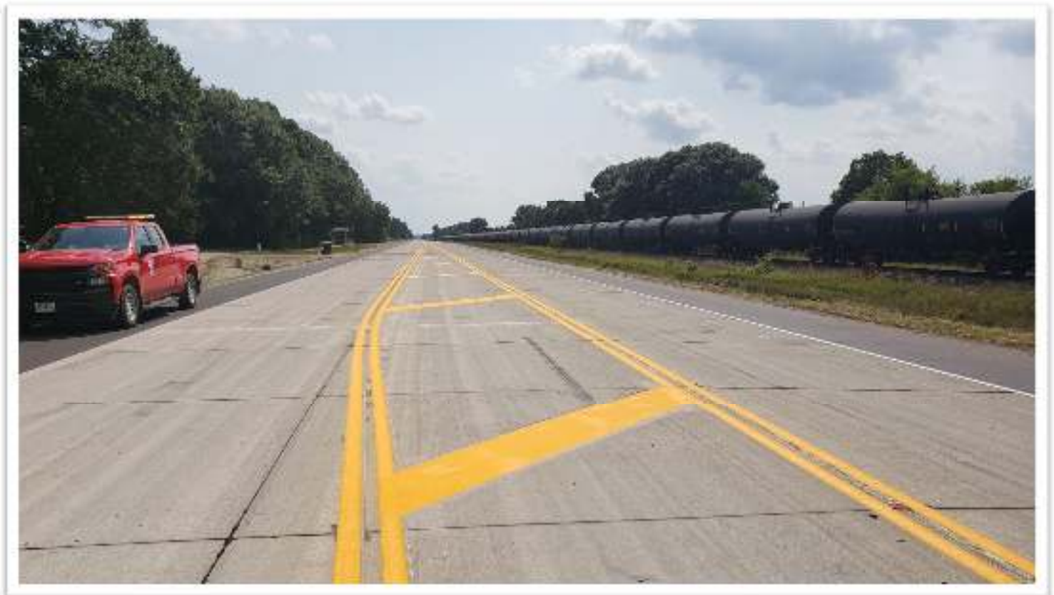
New permanent road markings.
