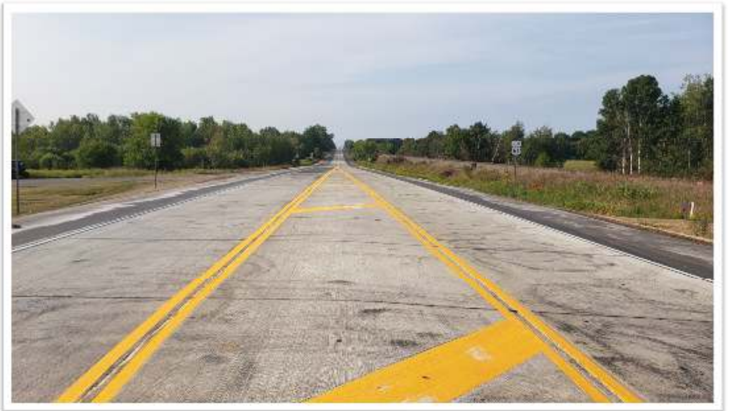
New permanent road markings.
