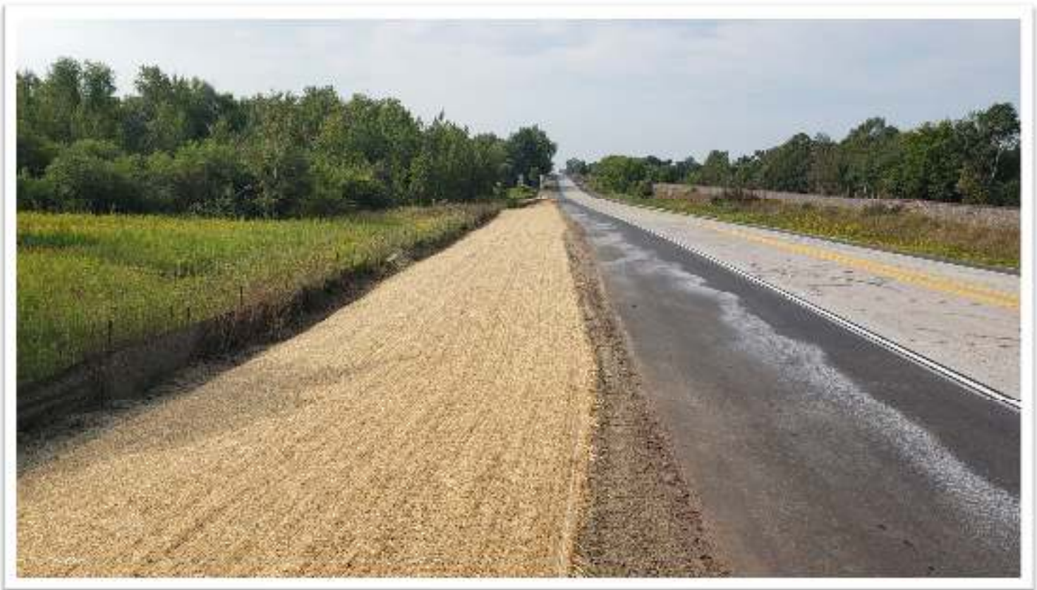
Seeded in-slope with erosion control blanket.
