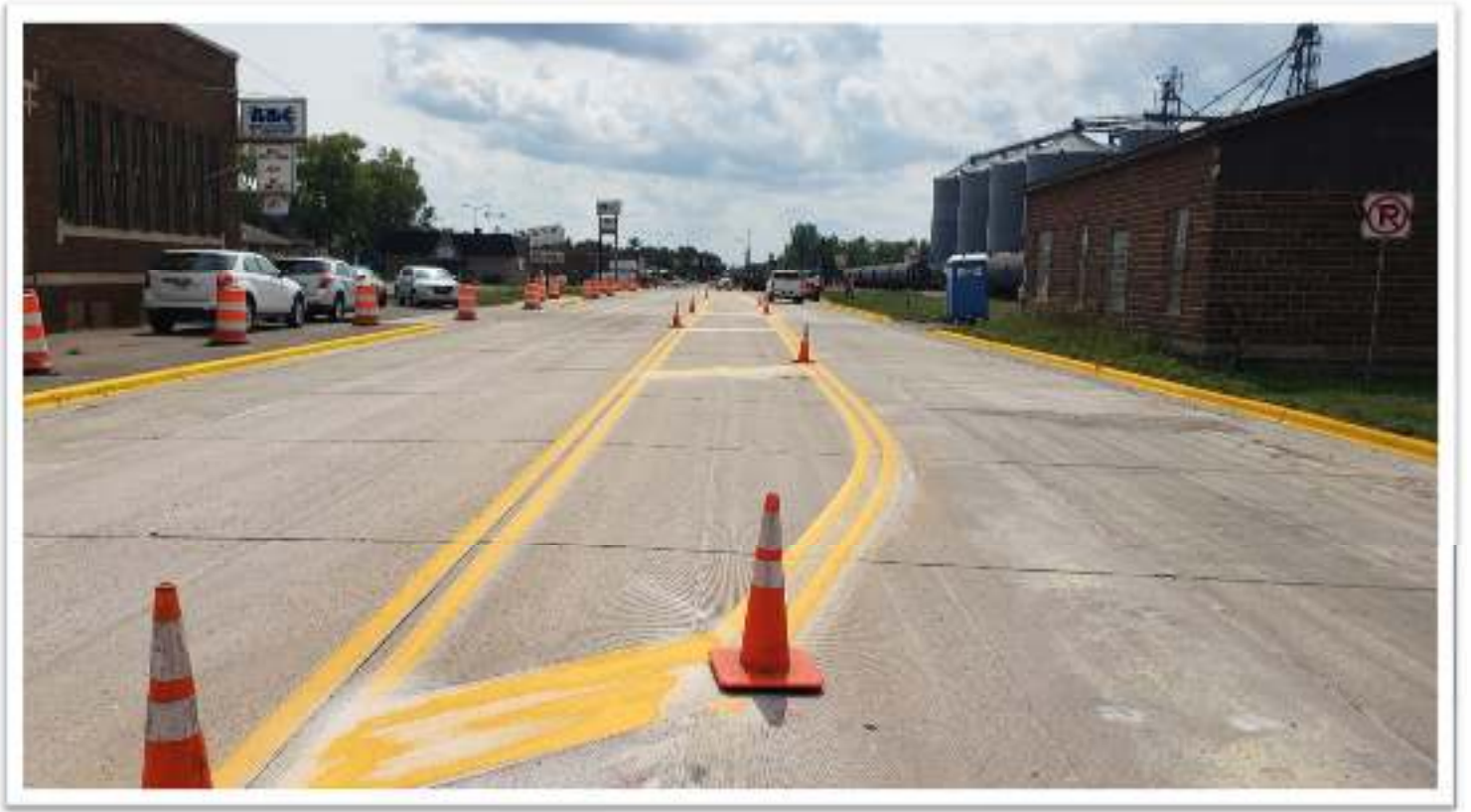
New permanent road markings.
