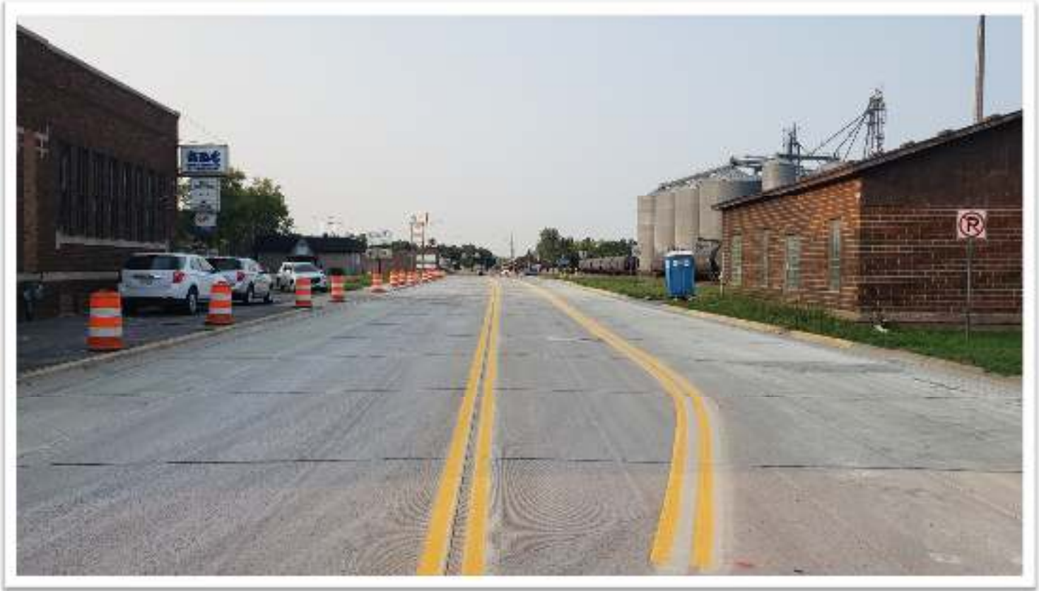
New permanent road markings.
