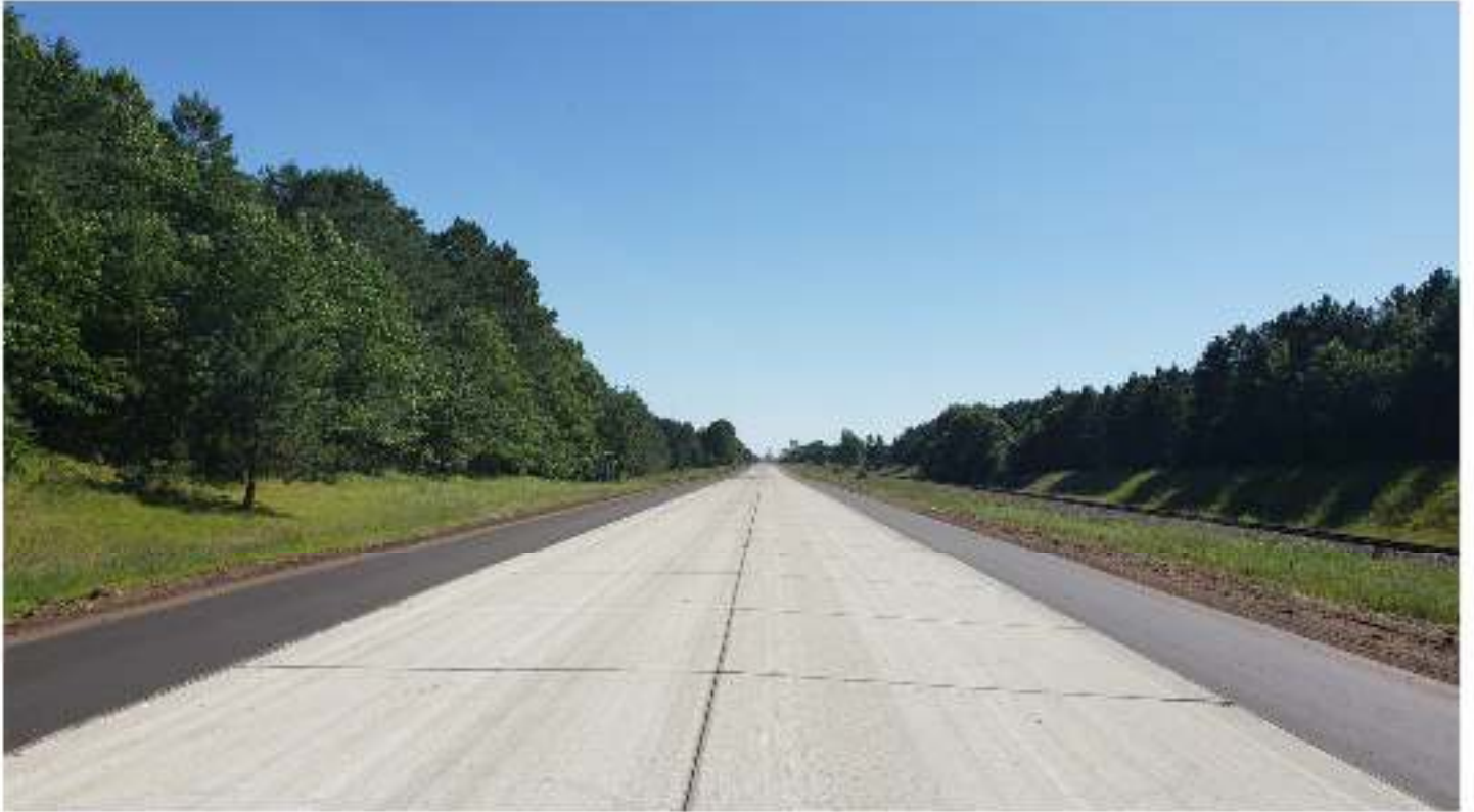
CSAH 30 before pavement markings.
