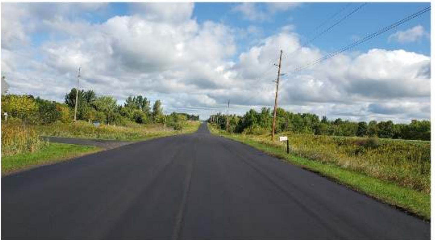
CSAH 4, newly paved surface.
