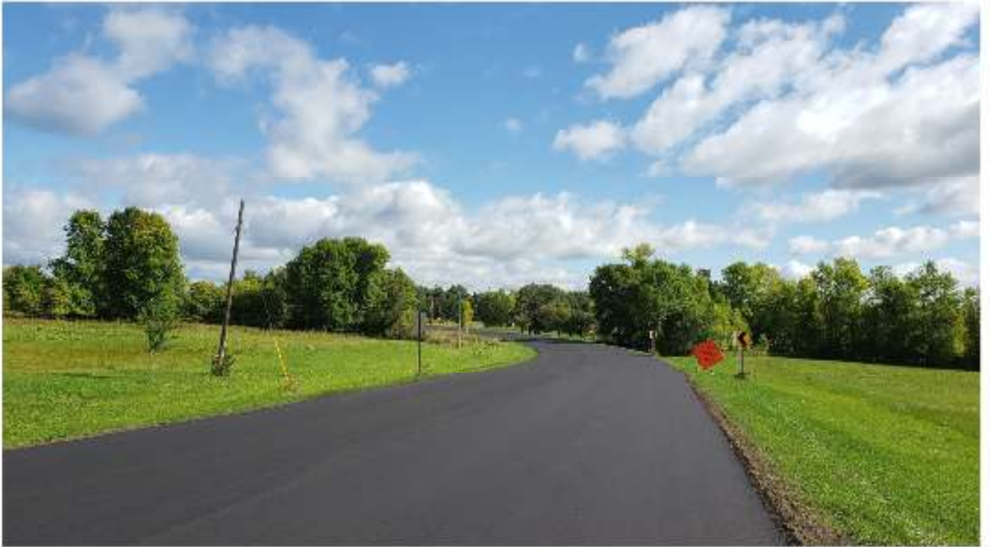
CSAH 4, newly paved surface.
