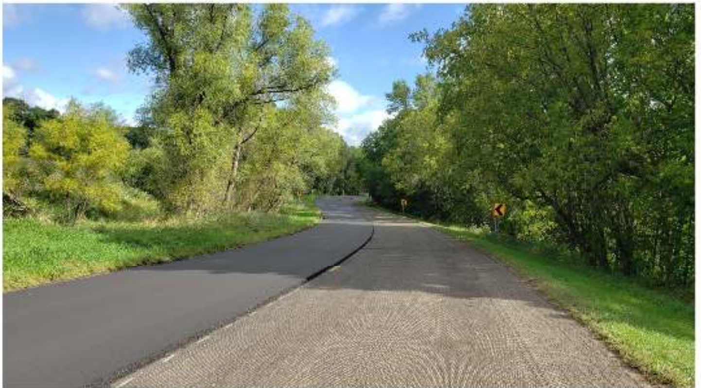
CSAH 4, new paved surface next to milled surface.
