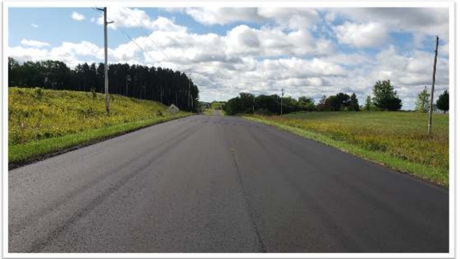
CSAH 4, newly paved surface.
