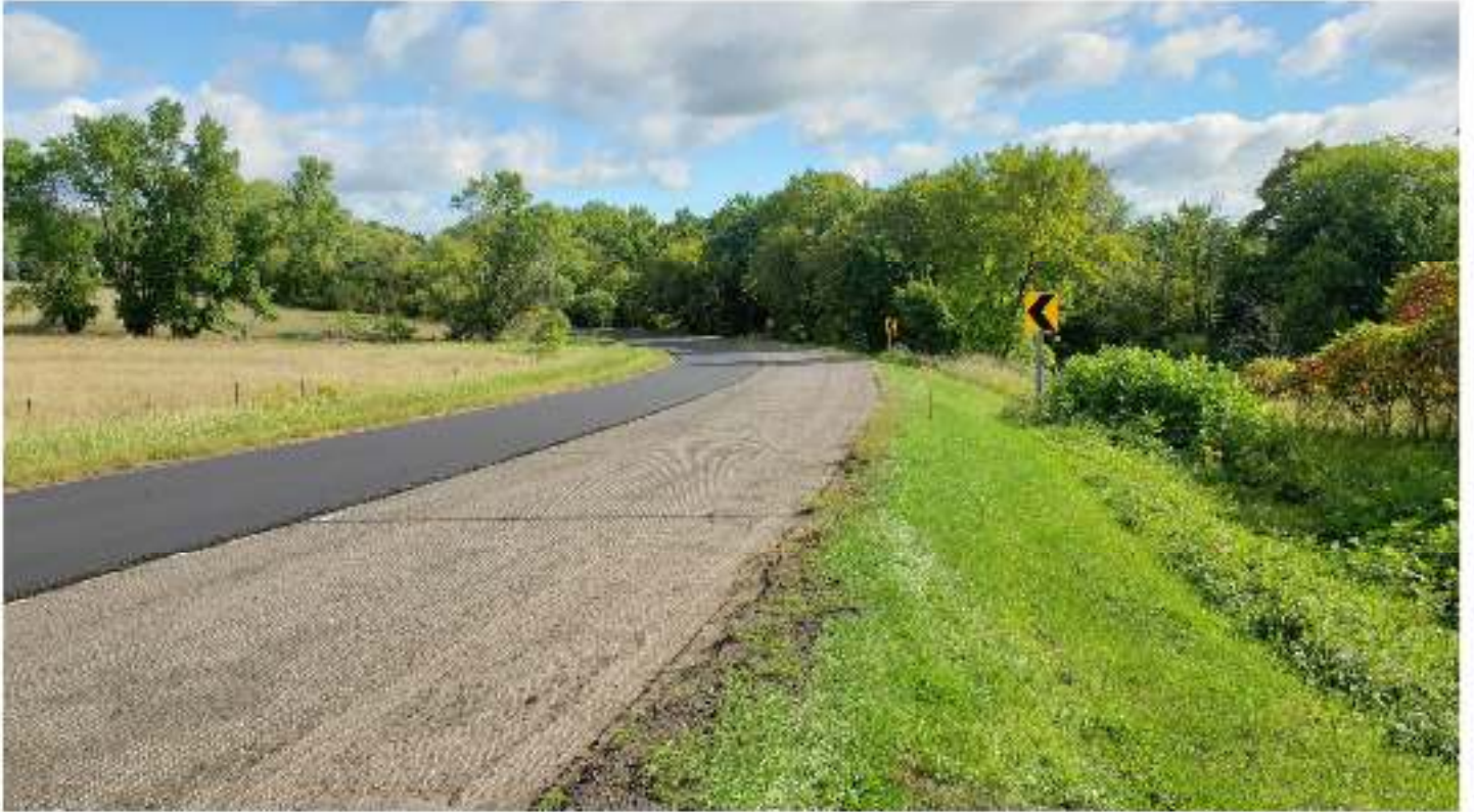
CSAH 4, Milled Surface next to new paved surface.
